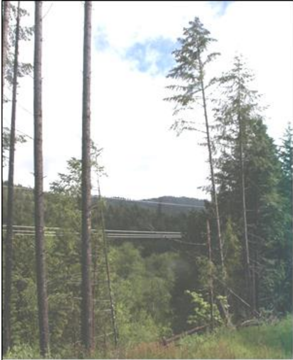
Figure 2-106. Unstable Trees Near Electric Lines Left after a Logging Operation
