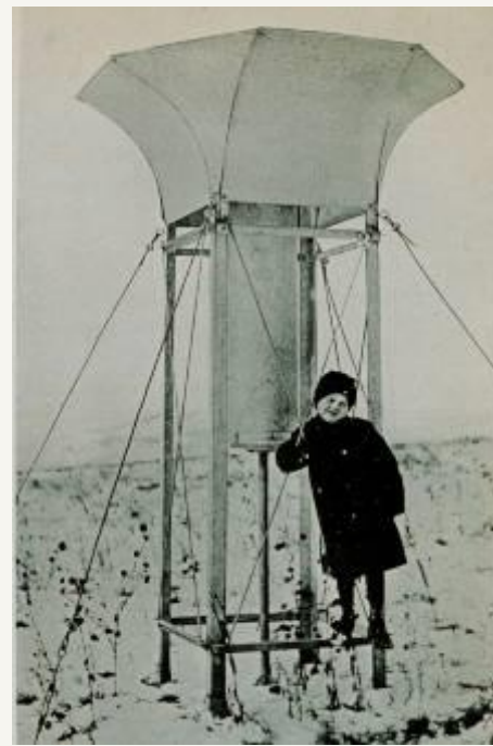
Figure 2-108. Shielded Snow Gauge Used in the Pacific Northwest to Register Snowfall, 1917
