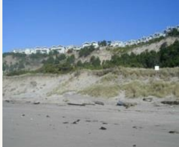
Figure 2-29. Erosion at The Capes Condominiums, Oceanside, Oregon
