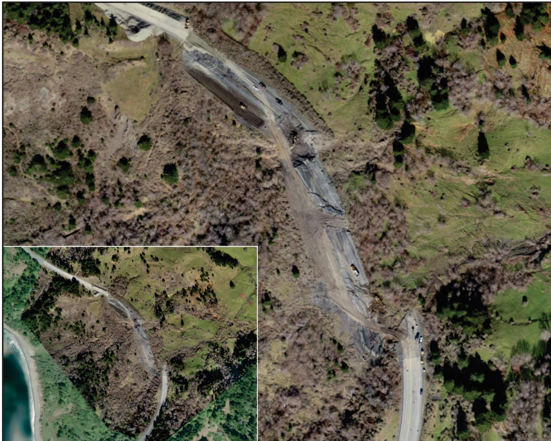
Figure 2-38. Landslide Movement Affecting U.S. Highway 101 at Hooskanaden Creek on March 3, 2019. Inset Photo Shows the Overall Scale of the Landslide and Its Proximity to the Coast
