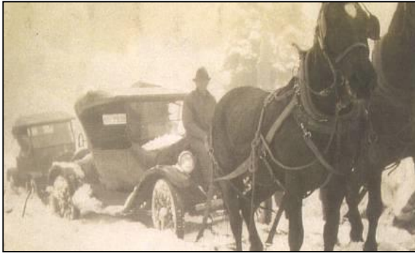
Figure 2-110. Rescuing Snowbound Vehicles, Old Oregon Trail Highway between Kamela and Meacham, 1923
