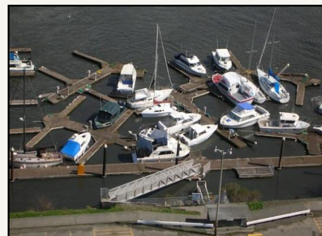
Figure 2-77. Tsunami Damage on the Chetco River, Oregon from the Tsunami Generated by an Earthquake Offshore Japan in 2011
