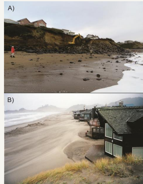
Figure 2-30. A) Emergency Riprap Being Placed in Front of a Home at Gleneden Beach, Following a Recent Bluff Failure (February 2013). B) Homes Being Inundated with Excess Sand during a Strong Wind Event in November 2001
