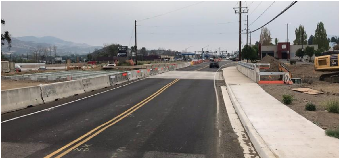
Exhibit 15: Coleman Creek Bridge - Under Construction (August 2022)
