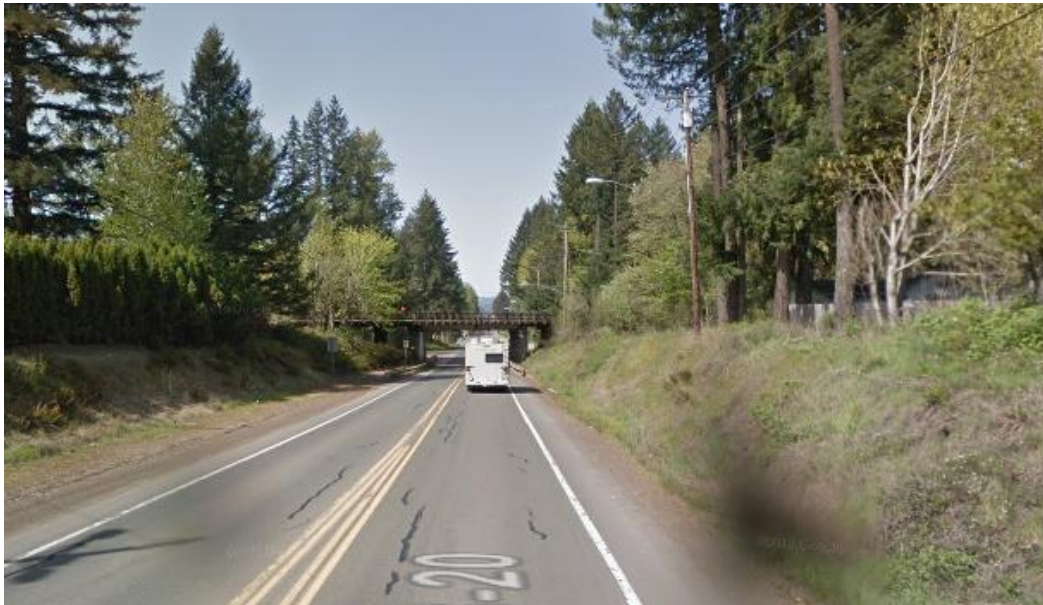
Bicyclists and Pedestrians forced to use edge of travel lane through railroad undercrossing.
