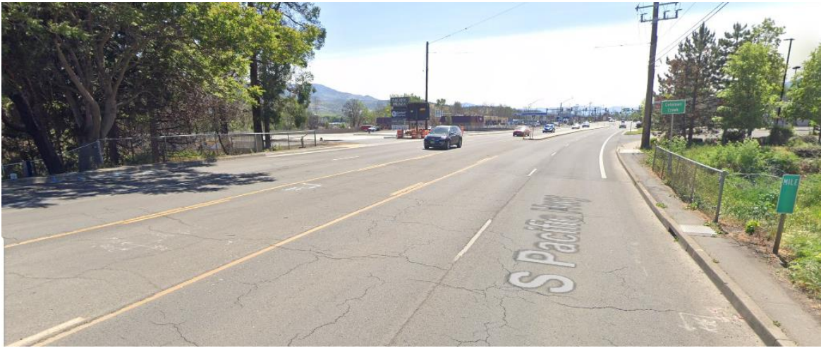
Exhibit 14: Coleman Creek Bridge - Before Project
