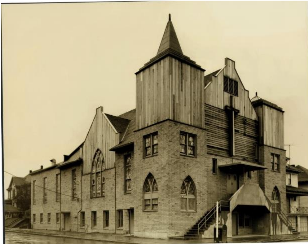
Vancouver Avenue First Baptist Church renovation. 1950-1959. Retrieved from the Digital Public Library of America, https://gallery.multcolib.org/node/4317 . (Accessed January 24, 2022.)
