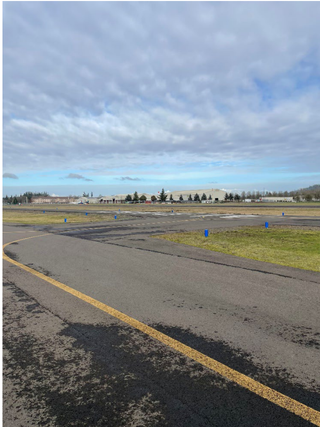
Taxi-Way Connector Realignment, Apron Rehab
