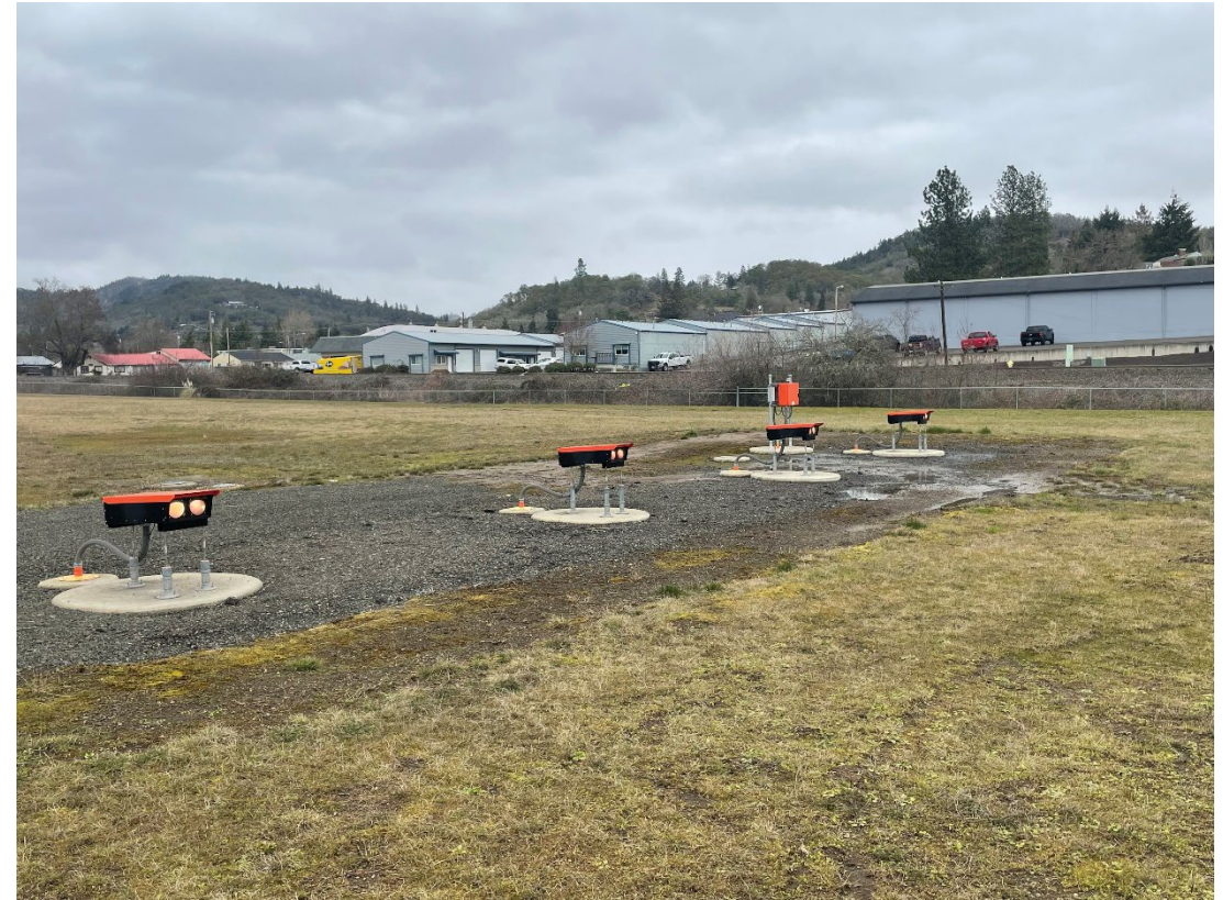
Runway 16 34 Lighting and Misc. Electrical Improvements
