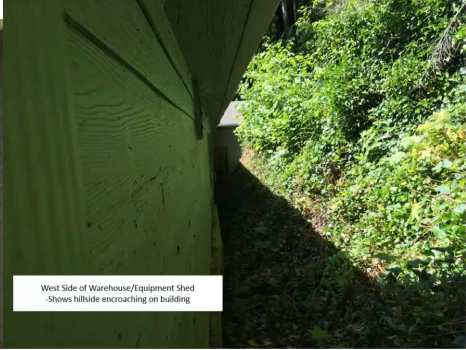
Northwest corner of Warehouse -Shows hillside encroaching on building. Have to dig it out every year.
