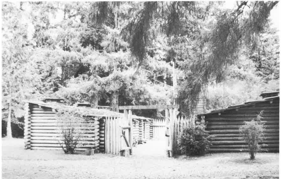
Oregon's first European-style building was Fort Clatsop, built by the Lewis and Clark expedition in 1805 as a winter shelter. It was abandoned the following year when the expedition returned east. This reproduction (based on a sketch in an expedition journal) was built in 1955 on, so far as can be determined, the original site. Fort Clatsop National Memorial is located off U. S. Highway 101 on Alternate 101, west of Astoria.
