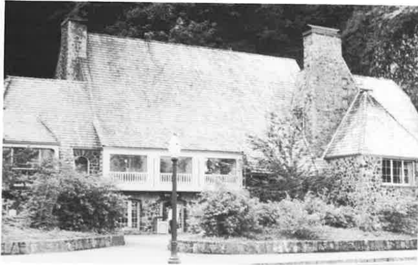
Public buildings don't have to be sterile and uninteresting. The lodge at Multnomah Falls is a case in point.
