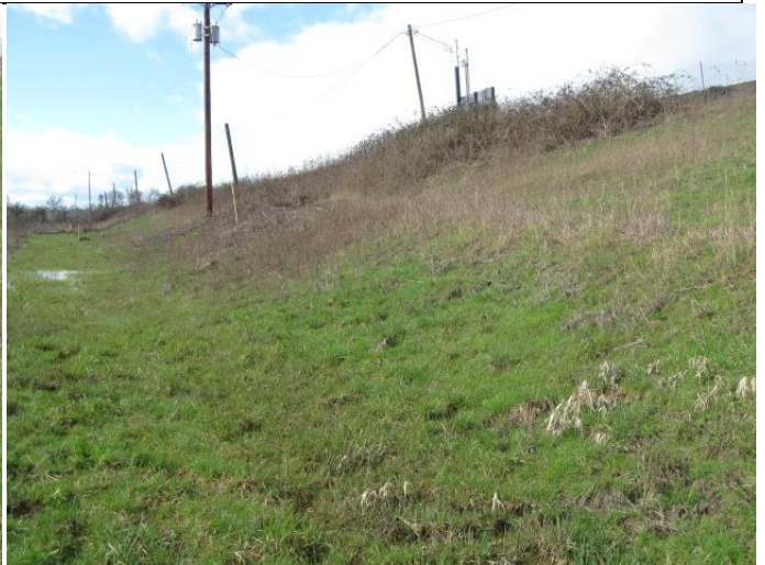
Southern perimeter berm (4 of 4).
