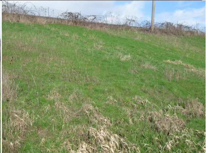
Southern perimeter berm (2 of 4).
