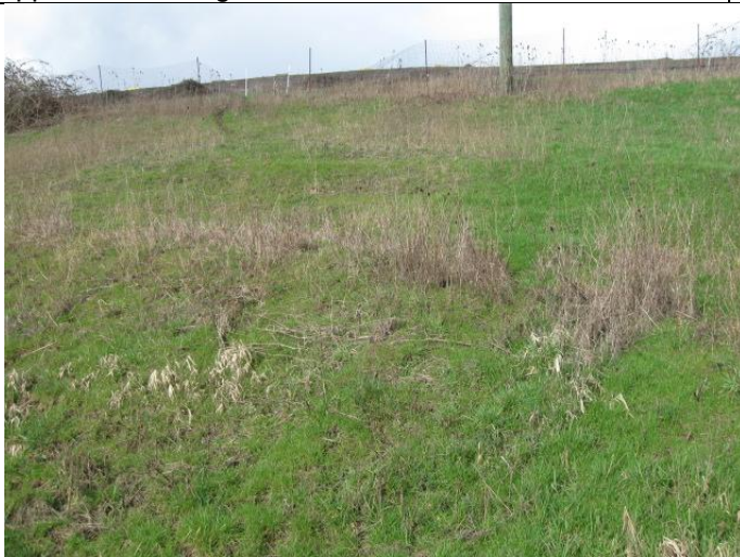
Southern perimeter berm (3 of 4).
