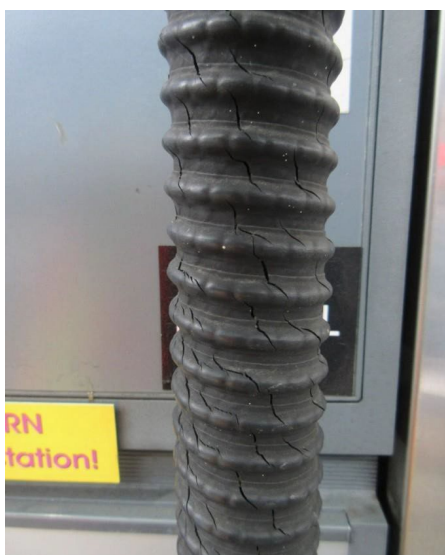
(AQGP-23) Balance System- Hose tears.
