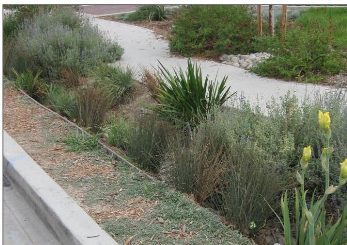
Capturing stormwater onsite through a bioswale, shown above, is effective and adds attractive landscaping features.
