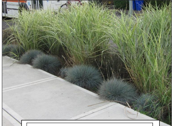
Capturing stormwater onsite through a bioswale, shown above, is effective and adds attractive landscaping features.
