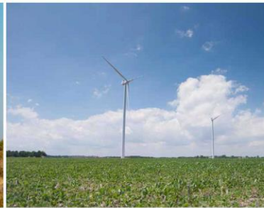
Port Dover & Nanticoke Wind
