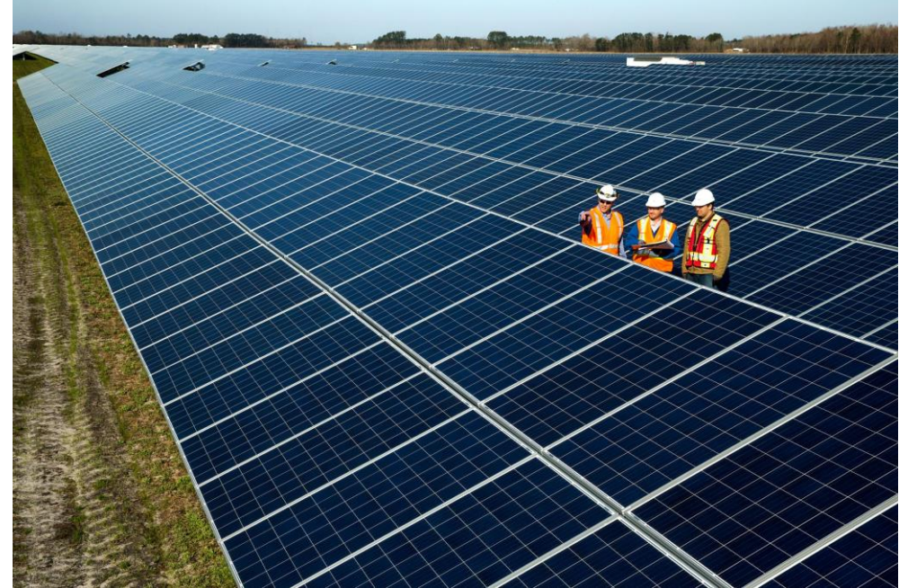
Capital Power's Beaufort Solar Facility, North Carolina
