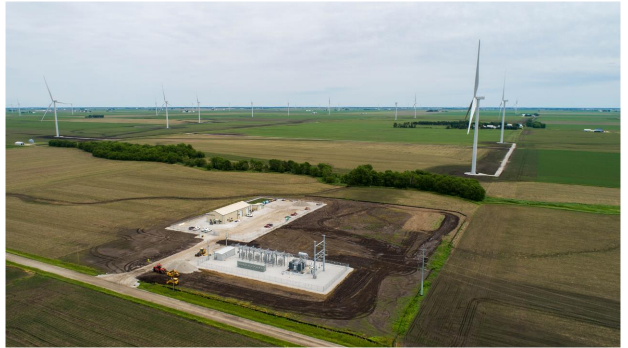
The operation and maintenance building at Capital Power's Cardinal Point Wind Energy Facility, Illinois.
