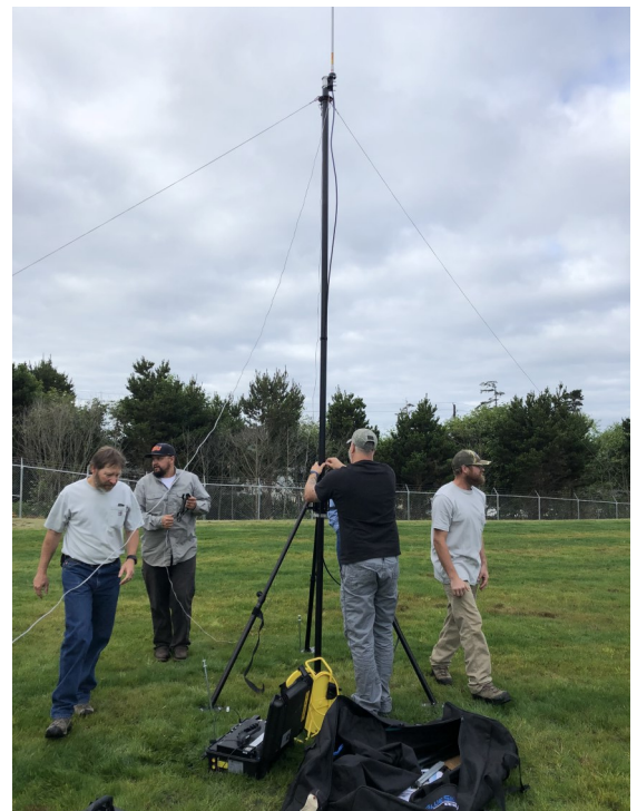
All CLPUD employees are trained to deploy the radio repeater system.
