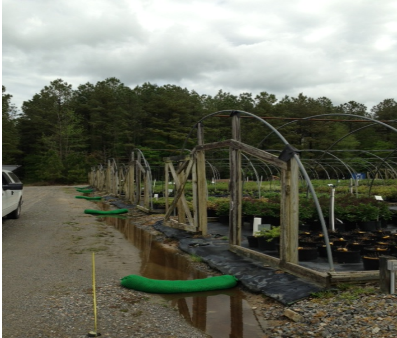
Image 3. Series of filter socks in sloped drainage ditch adjacent to hoop houses.
