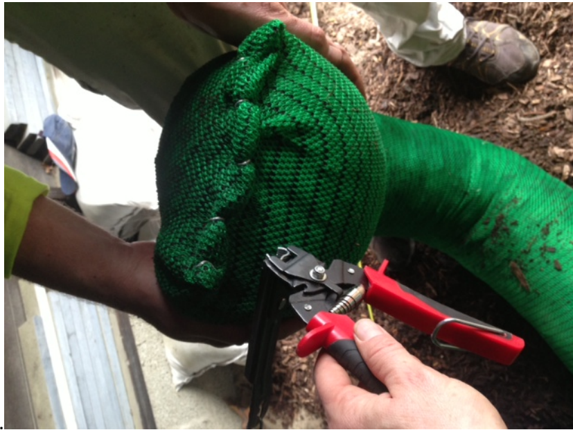
Image 2. Securing end of filter sock with c-rings
