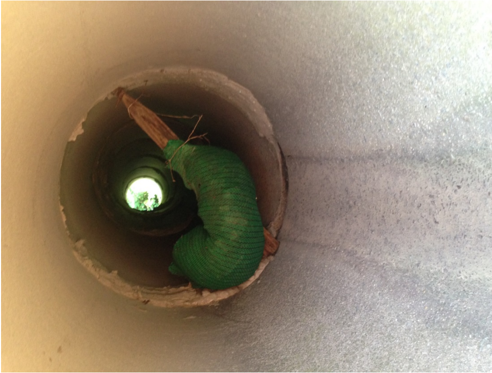
Image 5. Filter socks disturbed by storm event.
