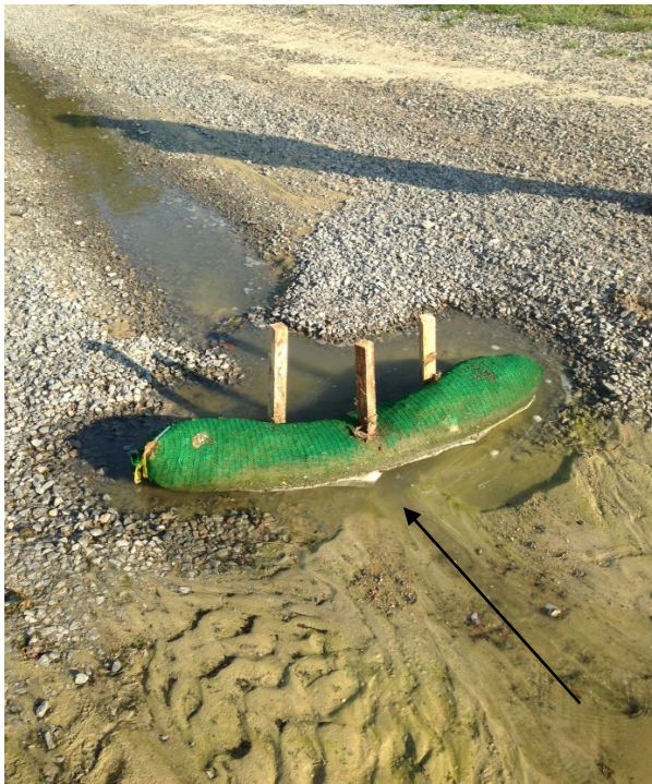
Image 6. Erosion around sock from storm event.
