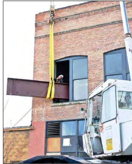
Workers carefully maneuver a steel beam into the Haskell Building
