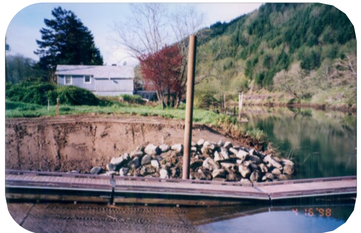
Riprap Stabilizing Bank below High Water Mark
