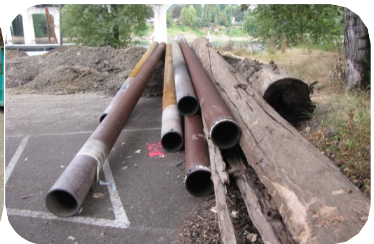
Steel Pilings and Untreated Woody Debris Collected for Reuse
