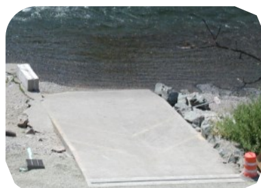
Newly built boat ramp
