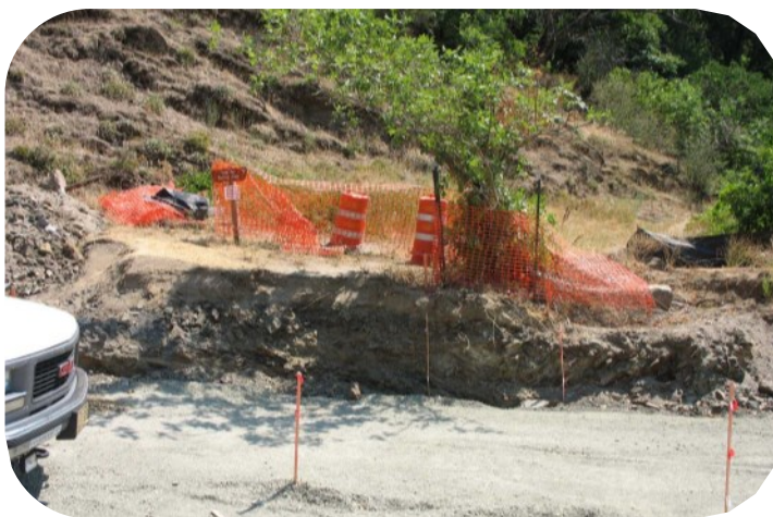
Protecting plants near worksite
