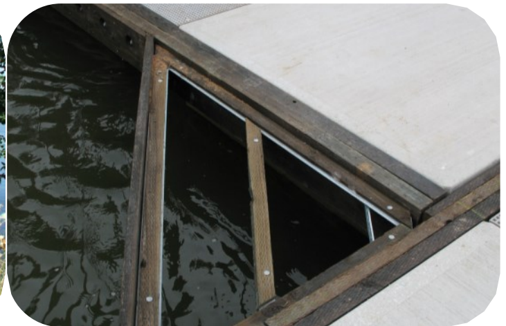
Concrete Docks Use Little Treated Wood
