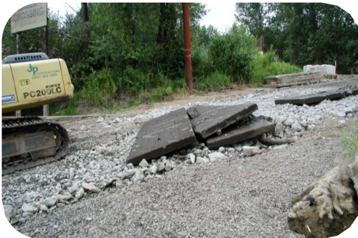
Removal of Whole Concrete Pieces
