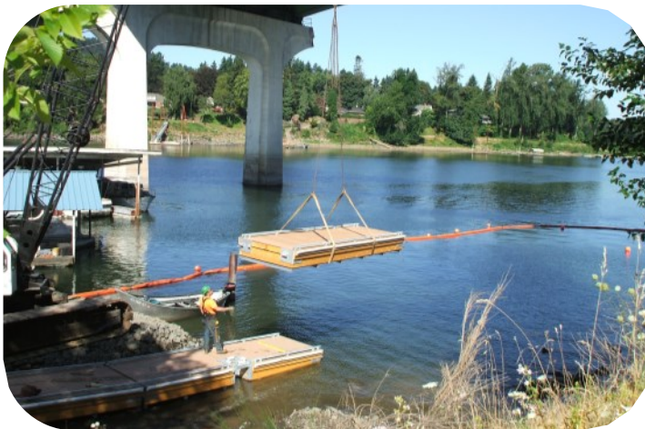
Installing Pre-fab Dock with Crane
