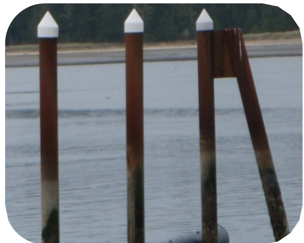
Figure 1. Pile Caps and Braced Piling
