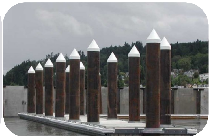
Piling Capped with Anti-Perching Devices
