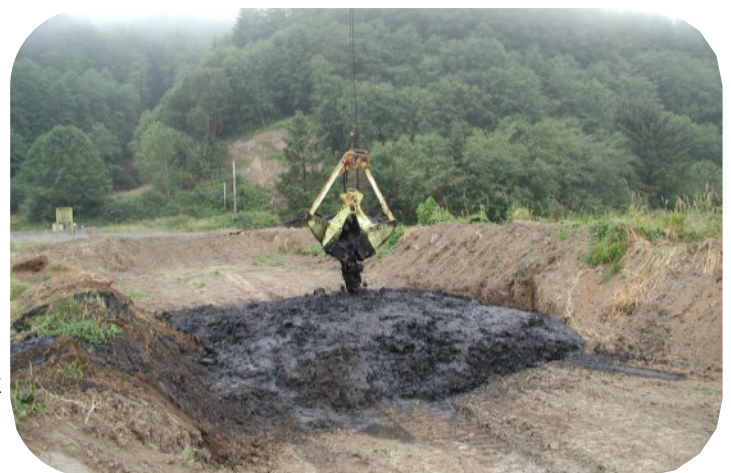
Properly Confined Dredge Spoils
