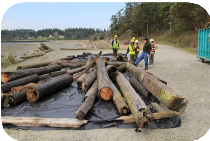
Creosote-Treated Debris on Plastic Liner Awaiting Removal to Hazardous Waste Facility
