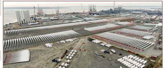
Example of Yard Storage Area for WTG components at Port of Esberg, Denmark Storage area approximately 2,000 feet in length
