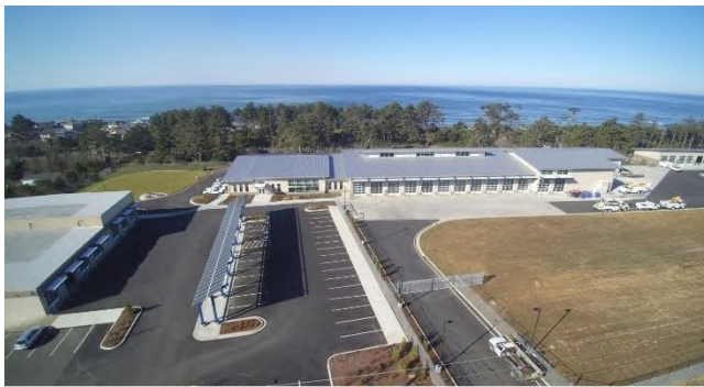
Central Lincoln People's Utility District in Newport built a seismically-sound operations center out of the tsunami zone.
