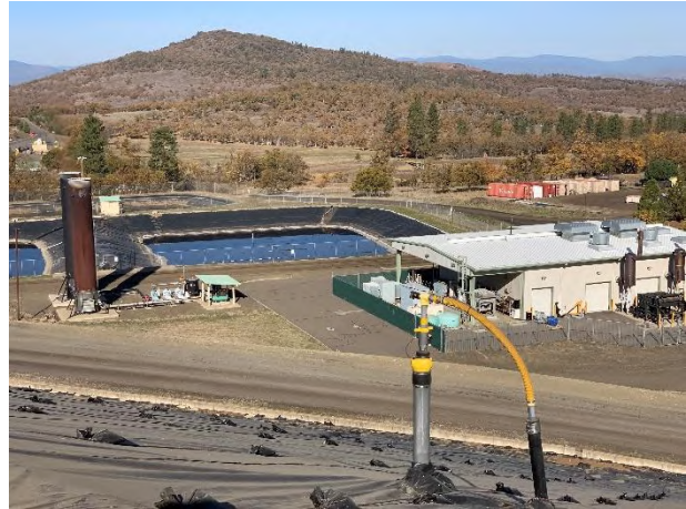
Landfill gas capture at Rogue Disposal and Recycling in Medford.
