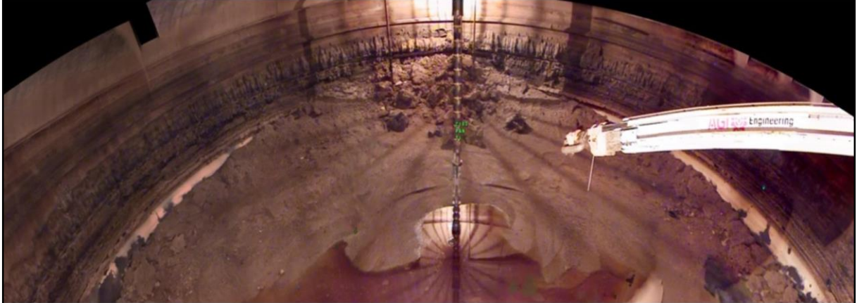
Tank C-102 – difficult sludge heel
