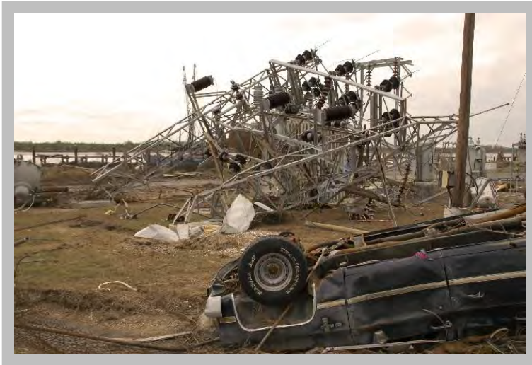
Figure 3.4: Hurricane Katrina Storm Surge – Electric Facility. Replacement of coastal power infrastructure based on 2012 capabilities may take one to three years for the Earthquake-only zone. (Source: FEMA.gov)
