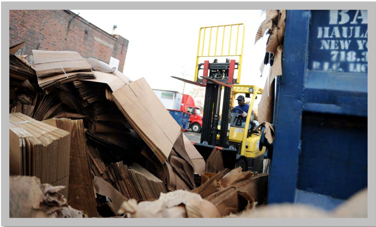
Figure 2.8: Brooklyn, N.Y., Dec. 4, 2012 -- Local Red Hook business, Cornell Paper and Box Company, continues cleanup of boxes at the warehouse that was flooded during Hurricane Sandy. (Source: Jocelyn Augustino/FEMA)
