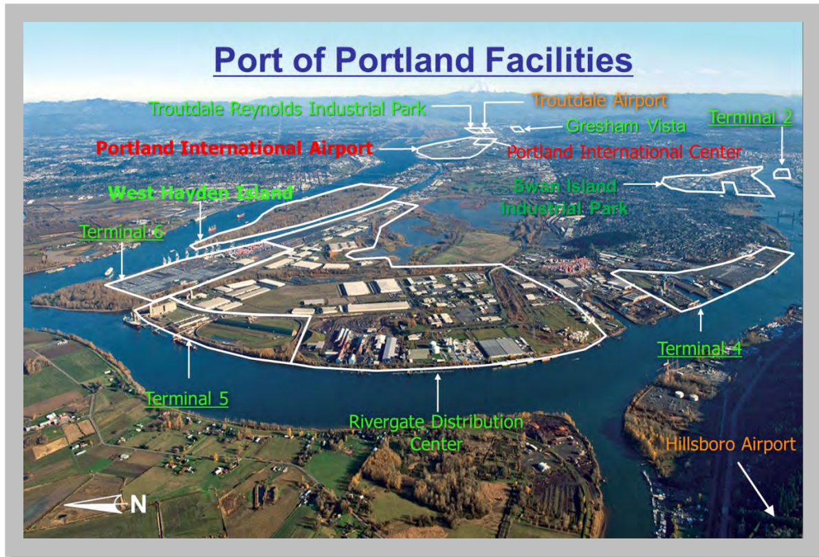
Figure 5.17: An aerial view of Port of Portland (Source: Port of Portland)
