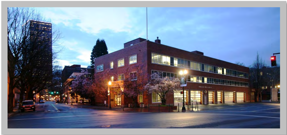
Figure 4.4: Some cities in Oregon have already started seismic rehabilitation program to strengthen the fire stations that are susceptible to serious damage in an earthquake. Fire Station #1, the largest in Portland, was retrofitted in 2009. It should now be in working order after an earthquake, serving downtown Portland. (Source: Peck Smiley Ettlin Architects)
