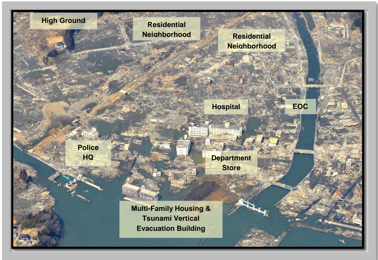
Figure 3.2: Critical Facilities in the Tsunami Zone – Minamisanriku, March 14, 2011. Because their hospital, emergency operation center, and other government and community service facilities were located in the tsunami inundation zone, the surviving community lost nearly all of its capacity to respond and implement recovery efforts. (Source: Asia Air Survey Co., Ltd.)
