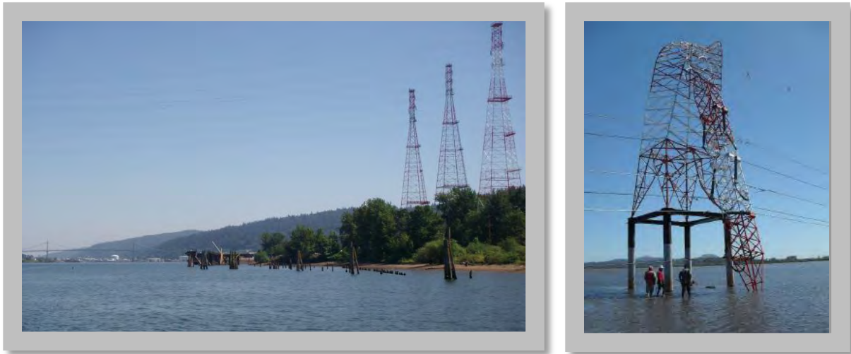
Figure 6.11 and 6.12: Left: These high voltage electrical transmission towers are built on a river bank in the CEI Hub susceptible to lateral spreading. (DOGAMI photo) Right: Structural damage to a high voltage transmission tower located at a river crossing in 2010 Chile earthquake. (ASCE Technical Council on Lifeline Earthquake Engineering – TCLEE)
