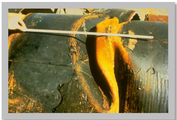
Figure 8.4: Welded steel pipe failed in compression, San Fernando (Sylmar) earthquake, California, 1971 (Source: Photo Source Unknown)
