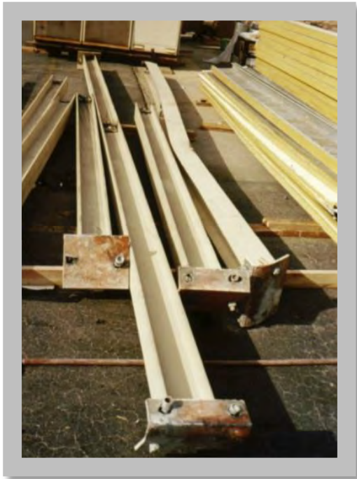
Figure 7.15 – Collection of damaged bracing beams removed from Central Office. Northridge earthquake, California, 1994. (Source: Alex Tang)
