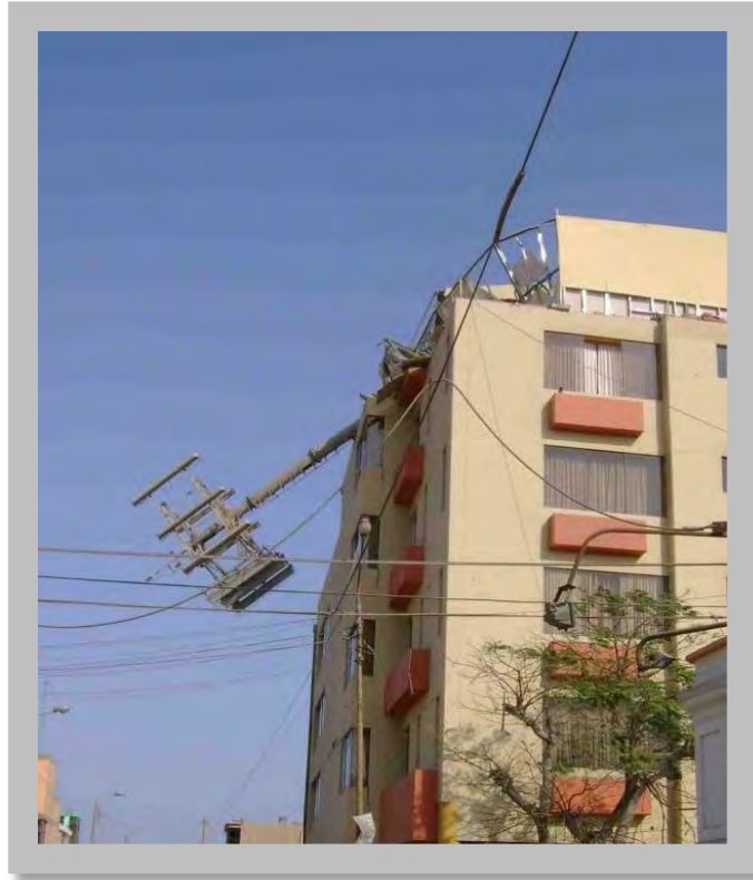
Figure 7.7: Cellular Base Station tower failure. This site is installed on the roof of an apartment building, which is not designed for critical infrastructure facility. Pisco, Peru earthquake, 2007. (Source: Alex Tang)
