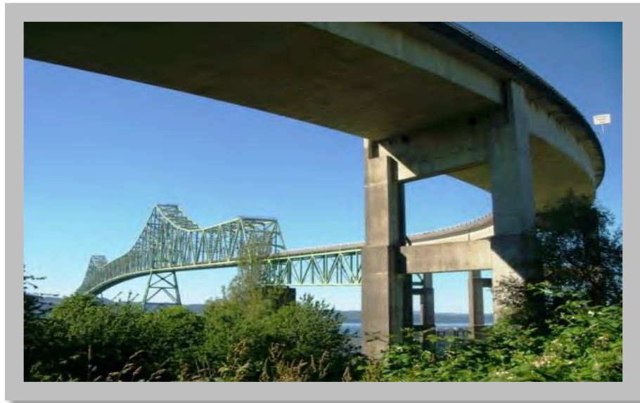
Figure 6.10: The approach (foreground) to the 1966 Astoria-Megler Bridge that spans the Columbia River has major structural deficiencies that could lead to a collapse following an earthquake. Damaged bridge sections could block waterway access to the CEI Hub. (DOGAMI photo)
