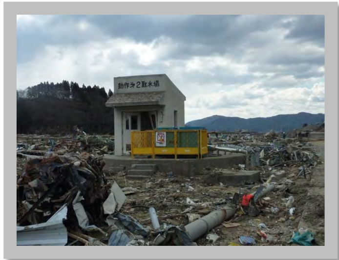
Figure 8.6: Water well and treatment facility in tsunami inundation area, Tohoku earthquake, Japan, 2011 (Source: Photo Source Unknown)
