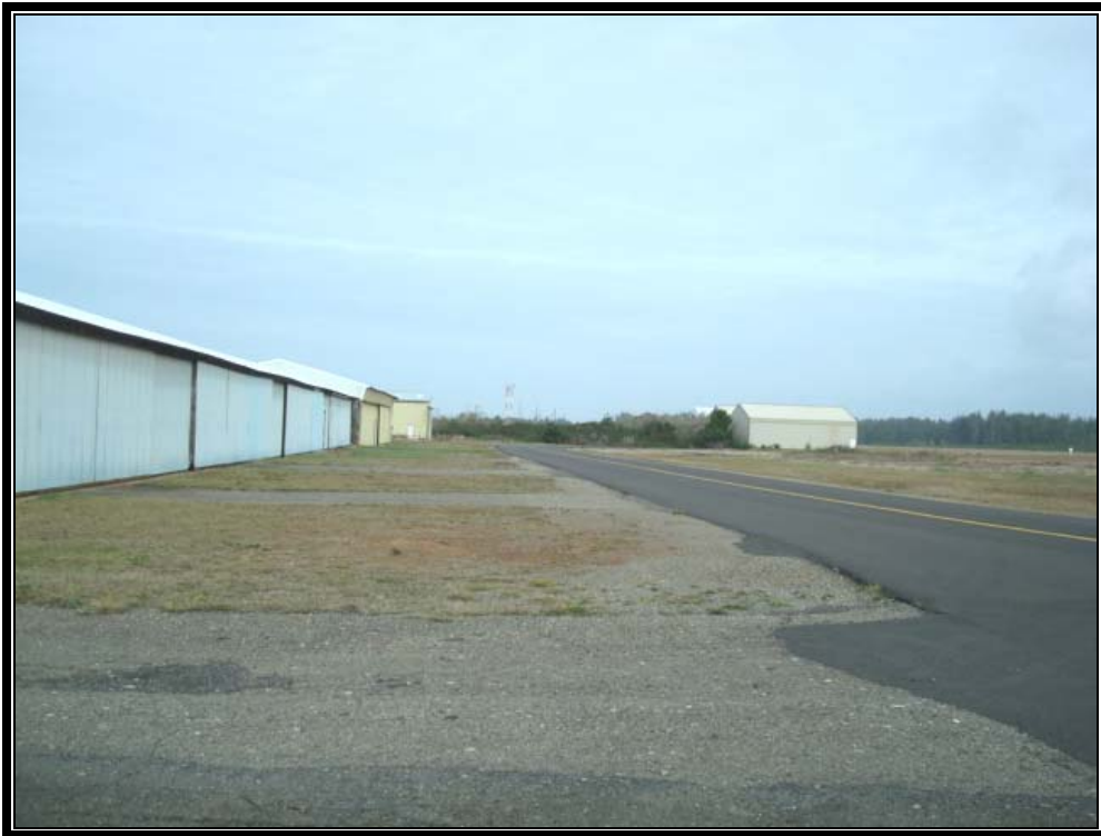
Viewing north from the ramp area.
