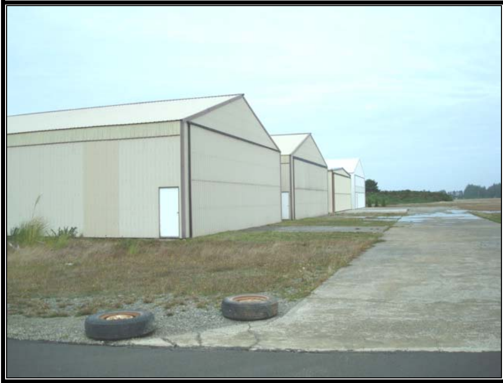
North hangar buildings, viewing north.
