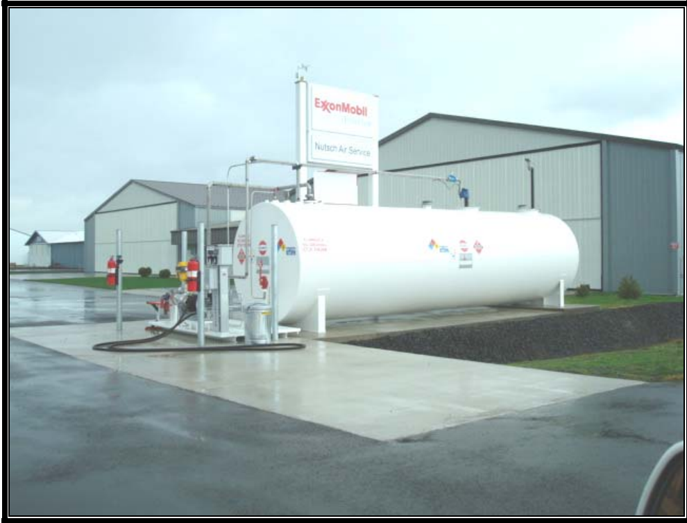
Fueling station and FBO building.
