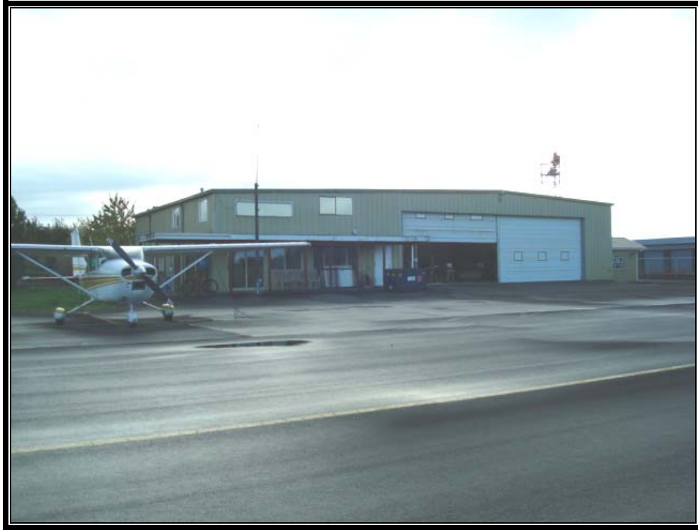
FBO building and ramp area.
