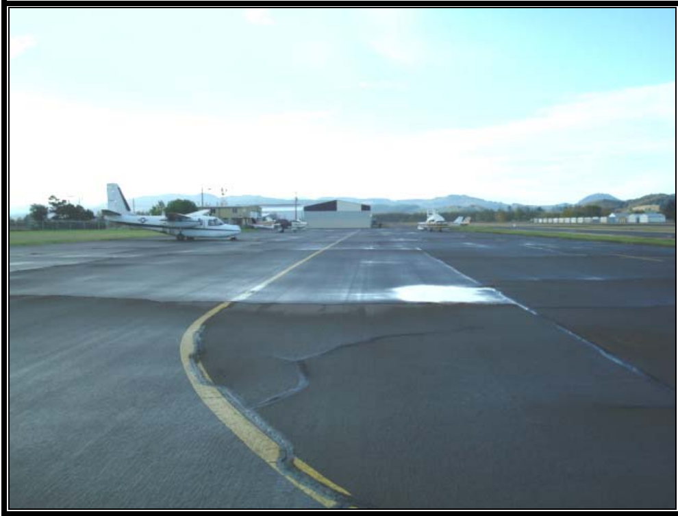
Viewing south at the ramp area.
