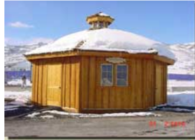
Wallowa Resources and partners built this kiosk from small diameter roundwood. The building served as an information center at the 2002 Winter Olympics.
