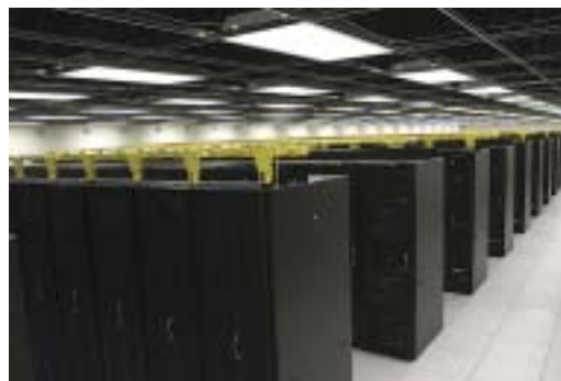
Yellow trays holding fiber optic cable run along the top of server racks
