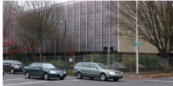
During construction, 7th Avenue and Pearl Street
