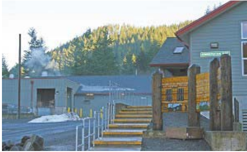
South Fork's administration building and inmate cabins sit in the hills of the Tillamook State Forest
