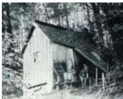
Flanagan house on South Slough
