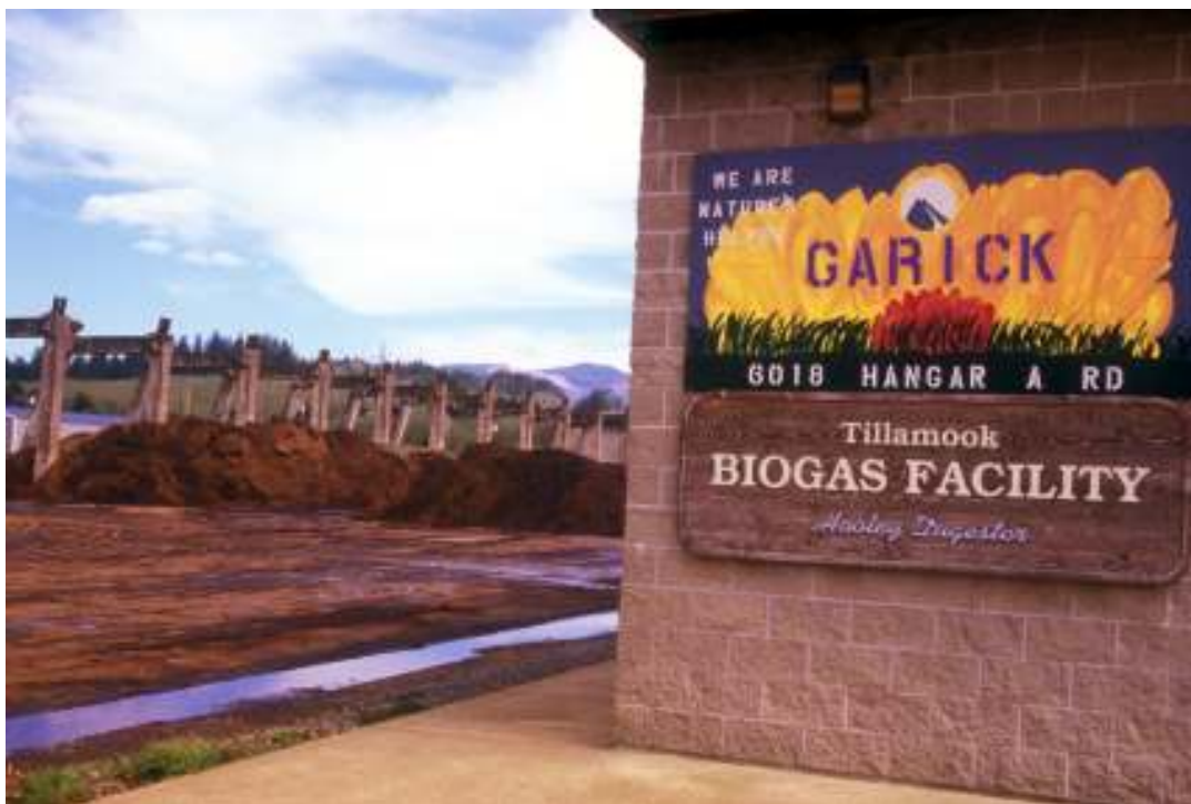
Tillamook Biogas Facility, Tillamook, OR
