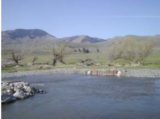
Completed Moore Diversion
