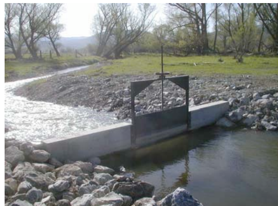
Moore Diversion head gate and concrete structure.
