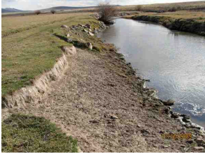
Compliance investigation: unacceptable streambank conditions cause by overgrazing
