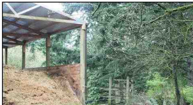
Manure storage facility implemented by landowner through assistance by the Tualatin SWCD
