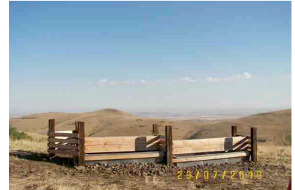
Watering facility that provides upland water for livestock, reducing grazing pressure near Butter Creek
