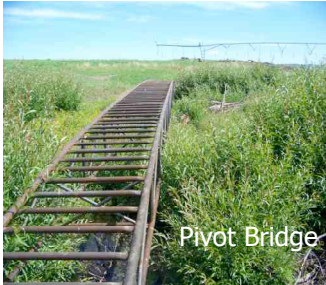
One of several bridges installed over Prairie Creek to allow for operation of a center pivot without contributing sediment to creek
