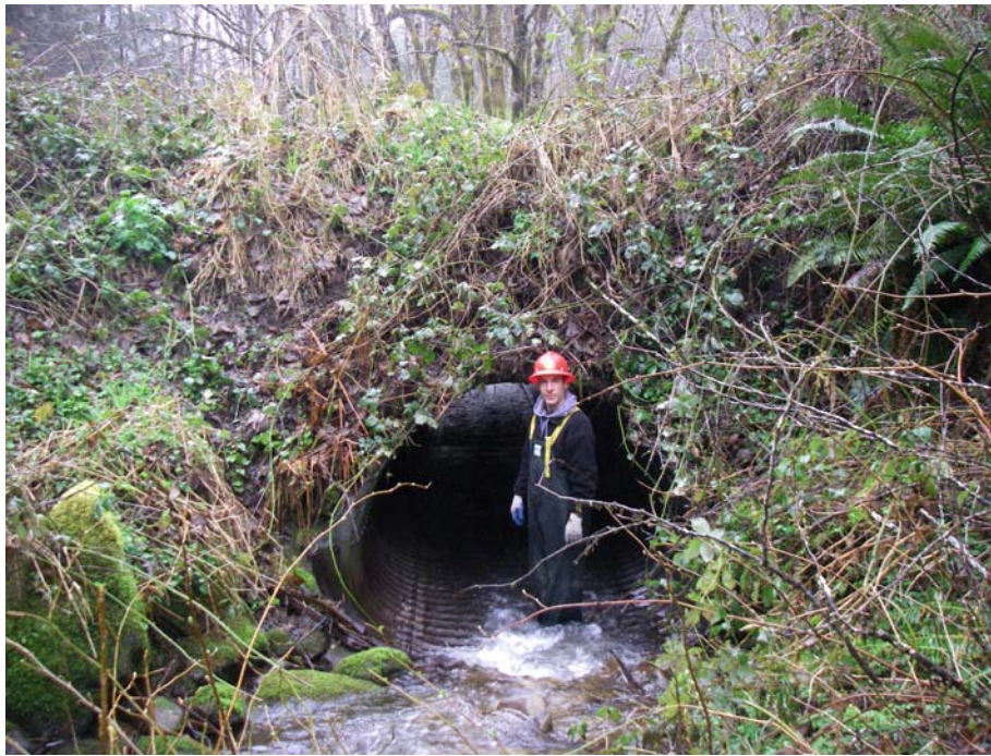
Before photo of Totten creek culvert.
