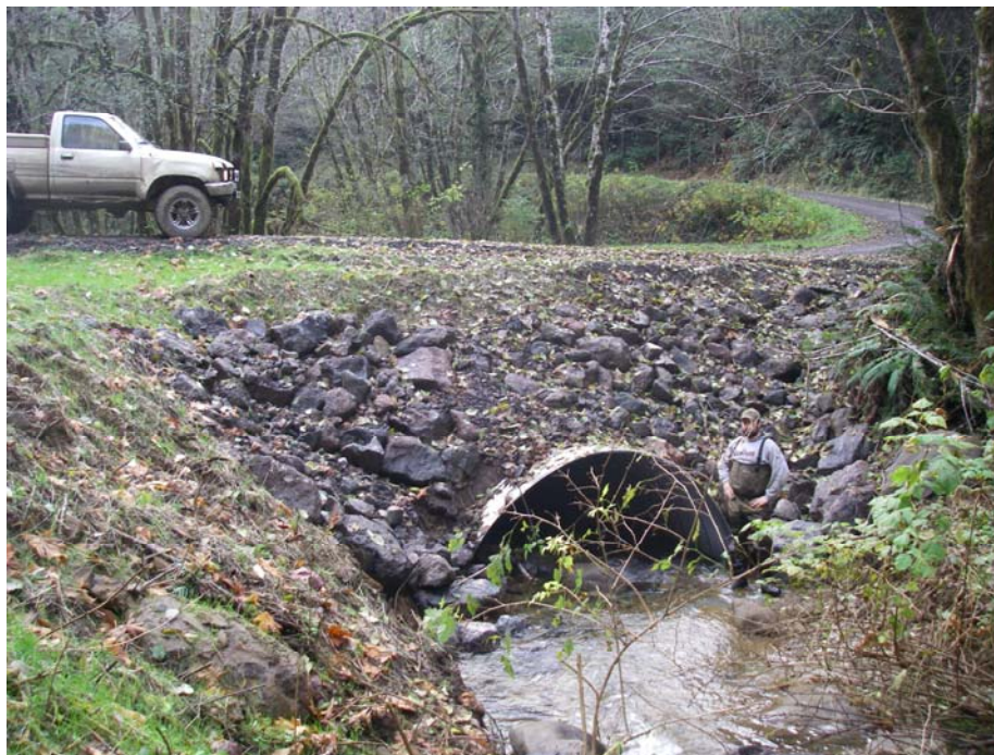
After photo of completed culvert on Totten creek.
