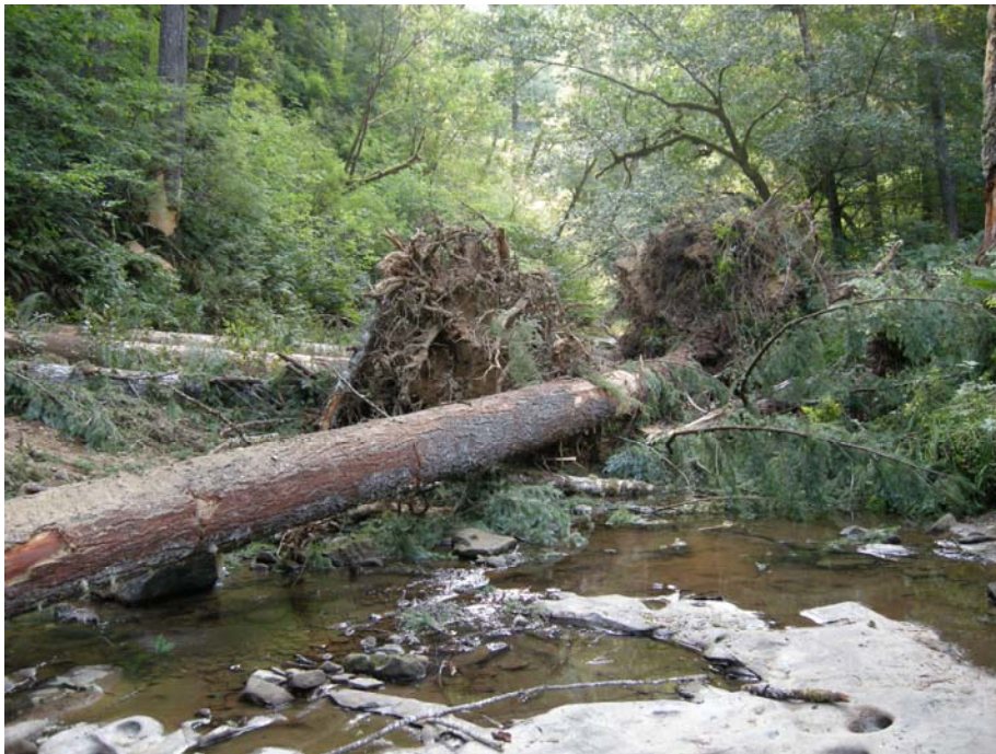
Completed structure of trees with rootwads in Elk Creek.
