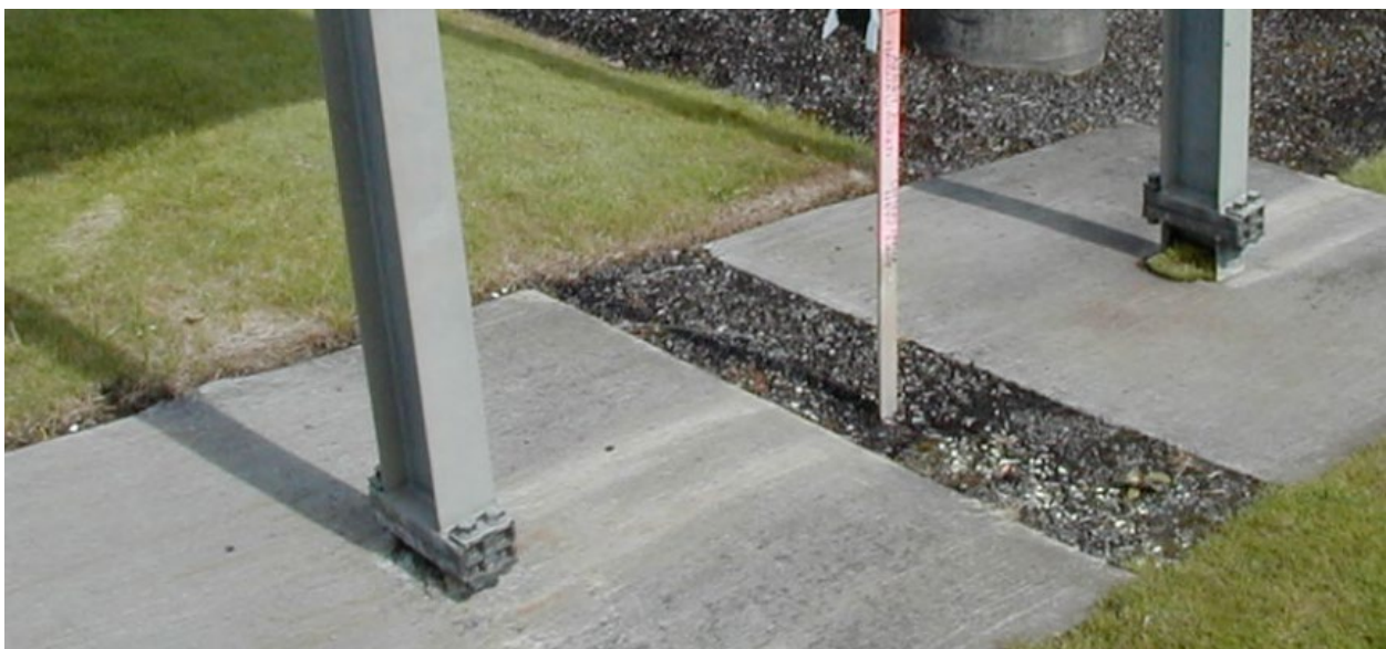
Figure 2: Multi-Post Breakaway Supports
