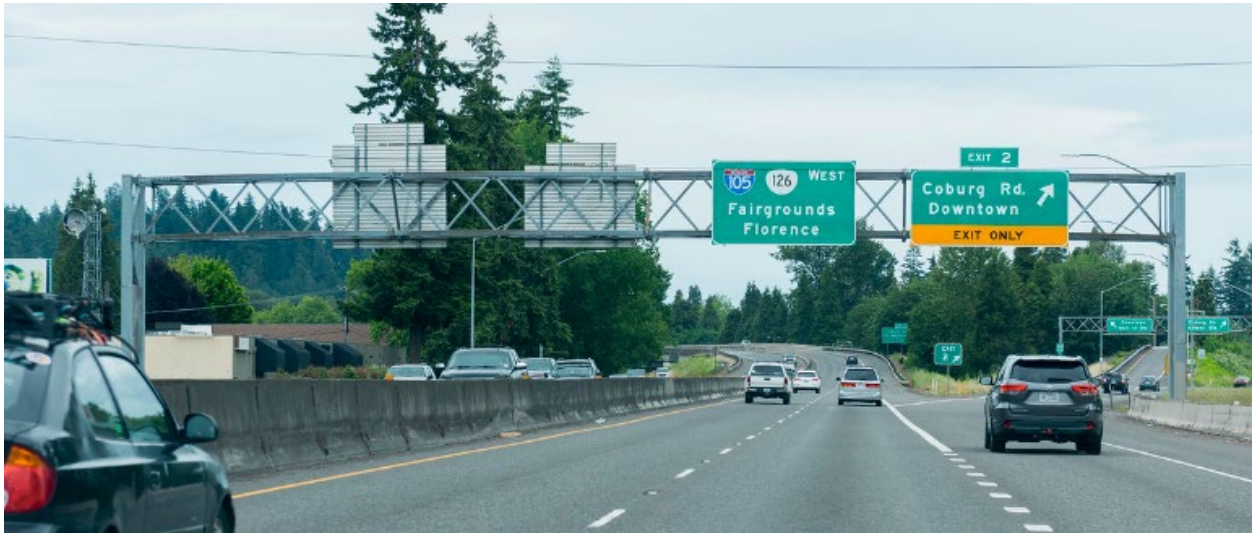
Figure 30: Sign truss bridge
