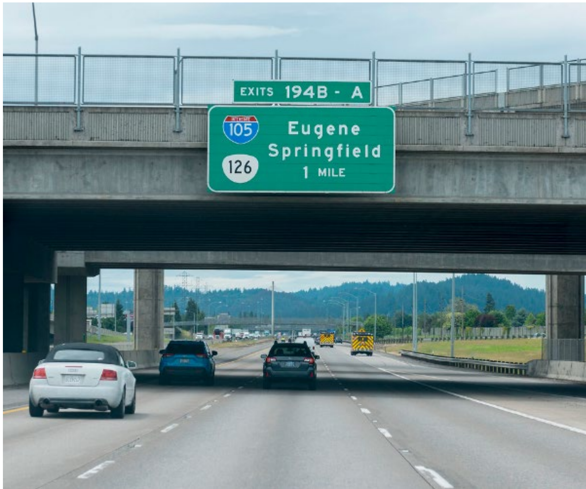
Figure 36: Sign mounted on the side of a bridge
