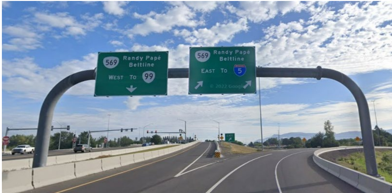
Figure 31: Monotube sign bridge
