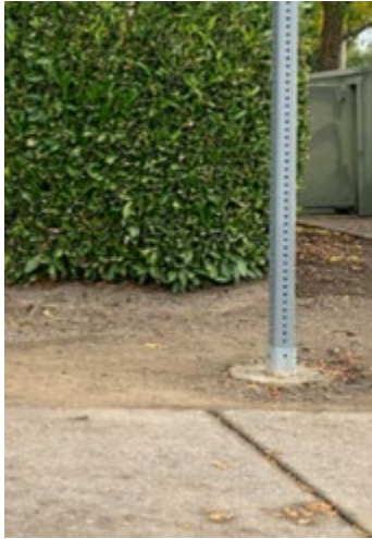
Figure 35: Anchor based perforated steel square tube sign support
