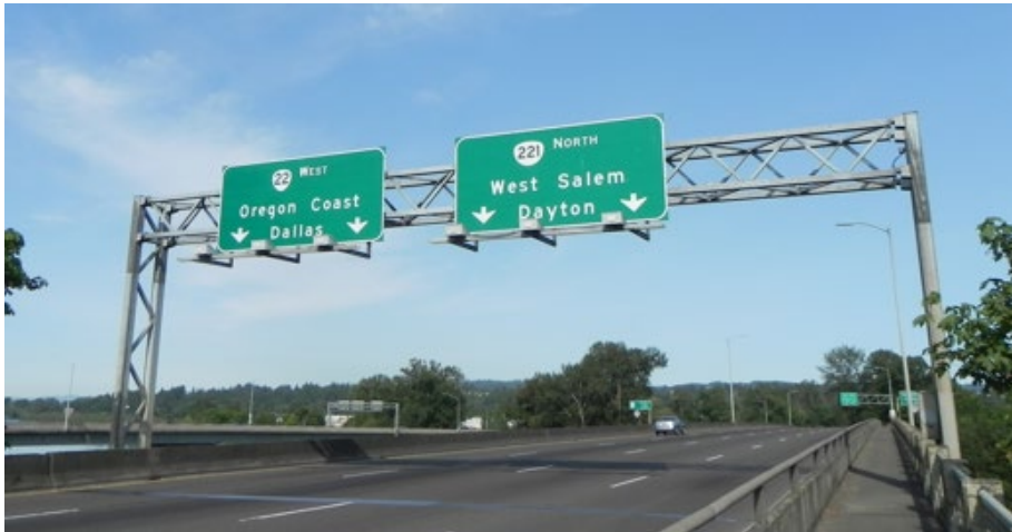
Figure 1: Truss Sign Bridge
