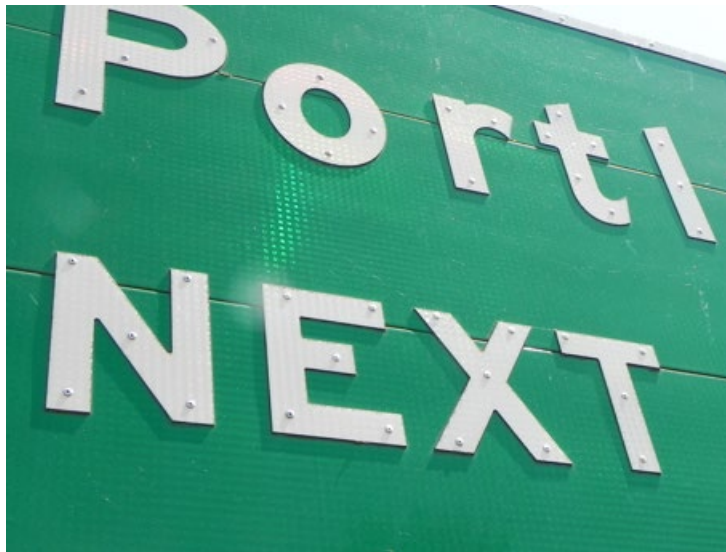
Figure 25: Demountable legend on extruded aluminum
