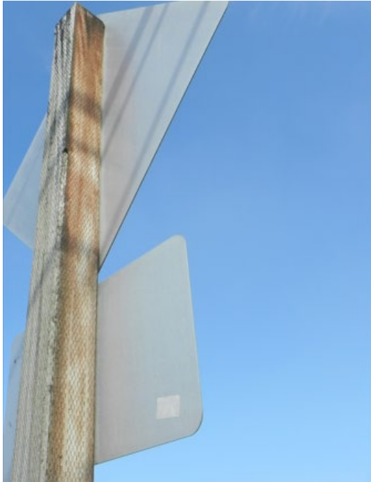
Figure 22: Sheet aluminum on a wooden post
