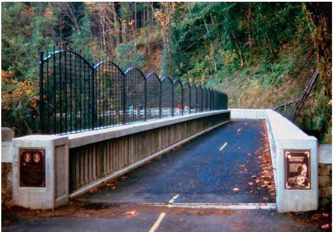
Figure 23—Toothrock Tunnel Bridge
