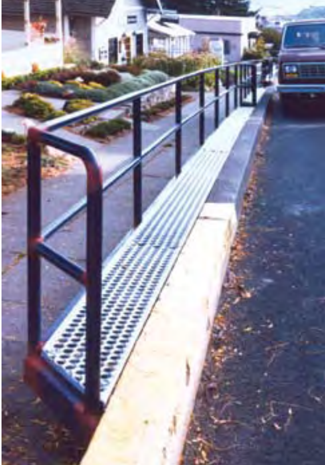
Figure 31—Pedestrian Railing in Hood River
