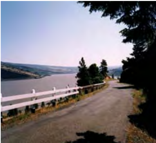
Figure 34—Restored Rubble Masonry Parapet Wall and Guardrail
