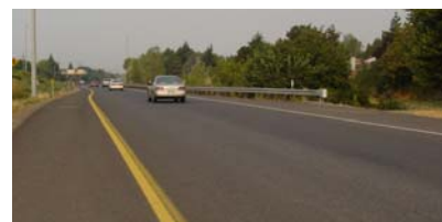
Westbound On-Ramp at Coburg Rd
