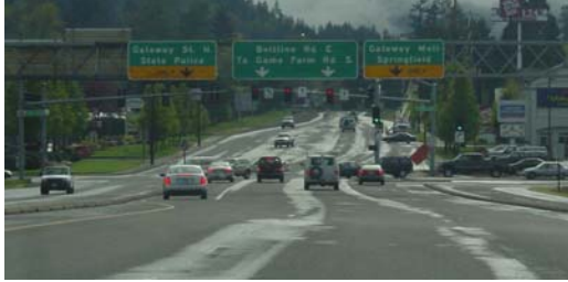
Eastbound Beltline Road at Gateway Street
