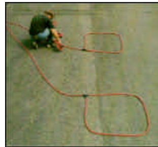
Figure 1-5 illustrates the location of the existing system detectors. The system detectors are used to collect traffic volume, speed and occupancy data. This data may be used for planning purposes, to identify fluctuations in traffic conditions or to implement traffic responsive timing plans.
