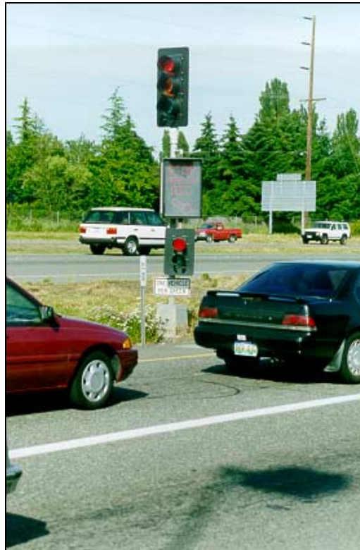
Ramp Metering Station
