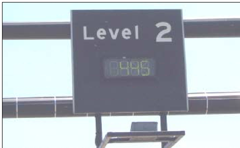
Sign providing parking space availability information by level source: Leigh Fisher Associates
