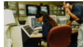
Operators use traffic monitoring and surveillance equipment to identify incidents and accidents.
