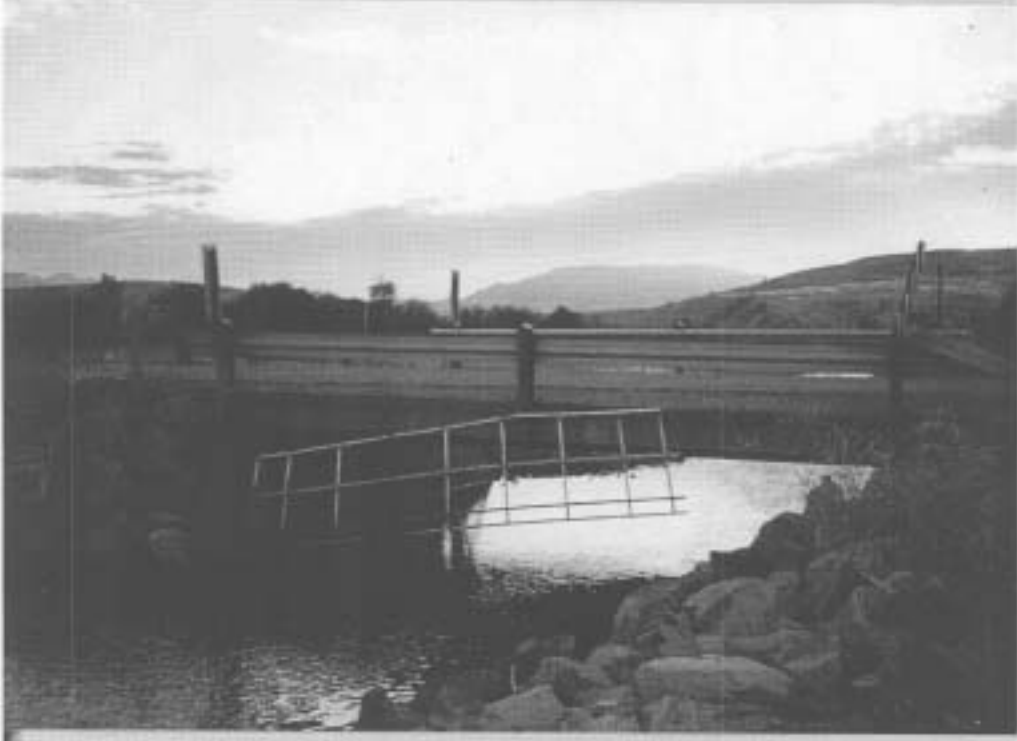
01C830 G:\PIWeb\local bridges\clear creek 01c830.doc
