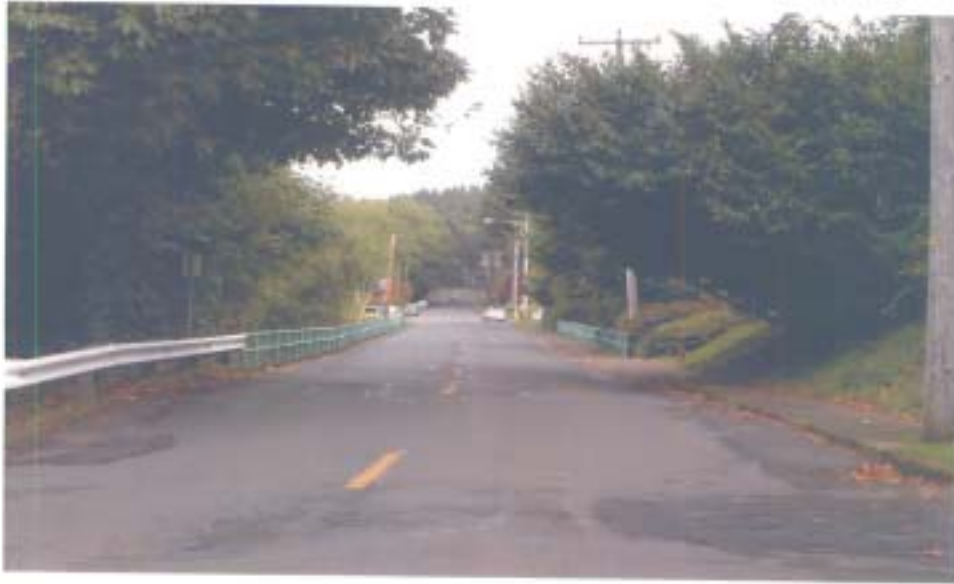
Photograph No. 1 — Approach looking east.
