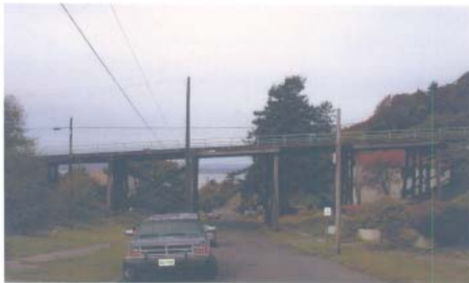
Photograph No. 4 — Elevation looking south.
