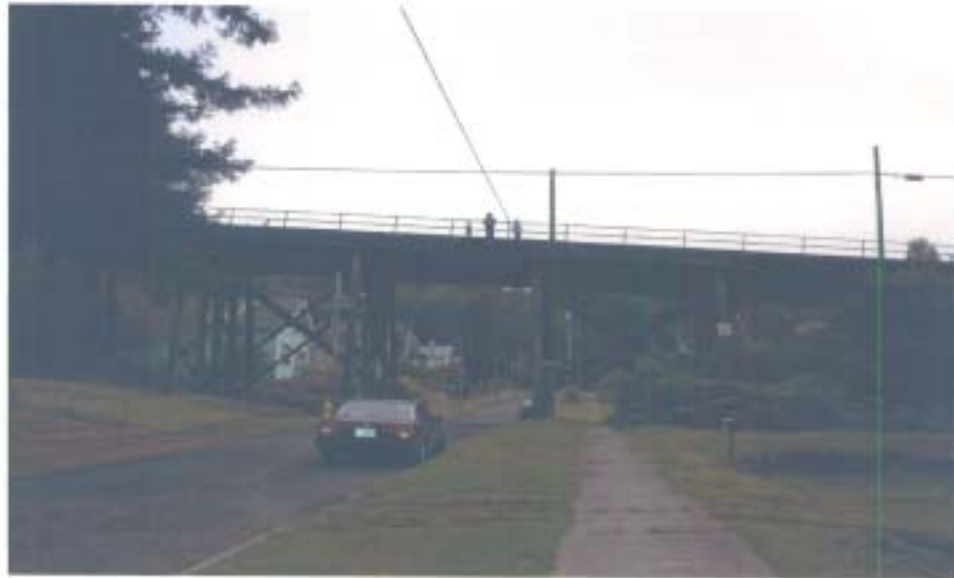
Photograph No. 3 — Elevation looking north.
