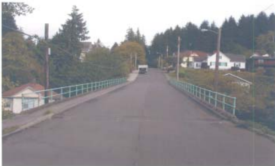
Photograph No. 2 — Approach looking east.
