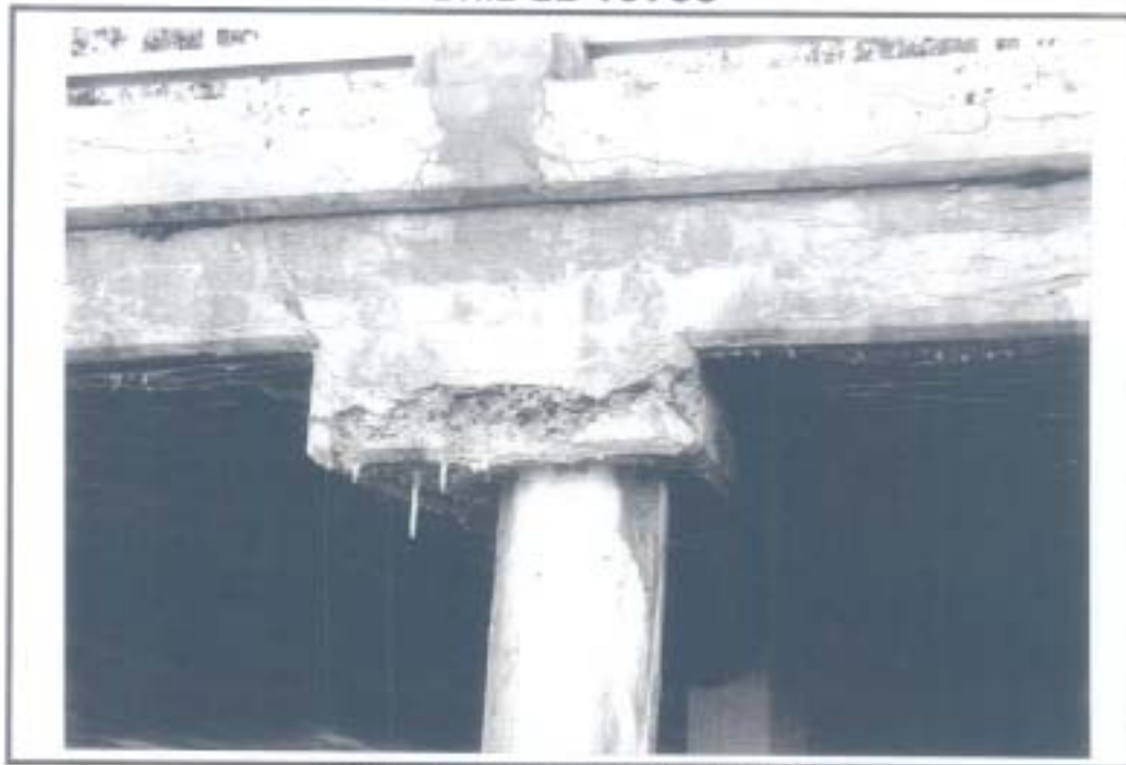
COLUMN UPSTREAM SIDE SOUTH OF MID SPAN
