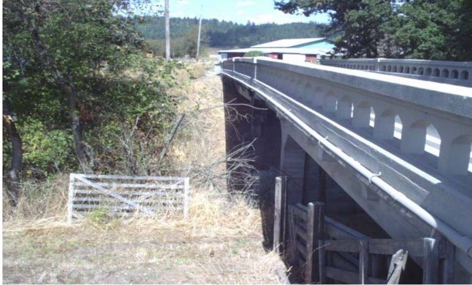
Photograph No. 9 — West side of bridge with utilities.
