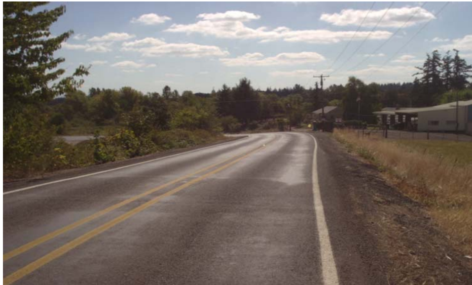
Photograph No. 4 — Substandard curve south of
