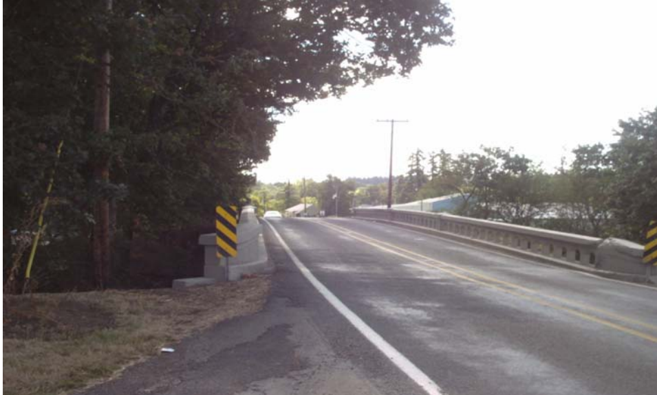
Photograph No. 1 — North bridge approach.
