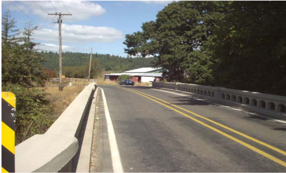
Photograph No. 5 — Bridge deck.
