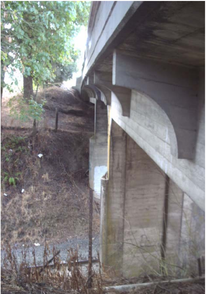
Photograph No. 7 — East side of bridge
