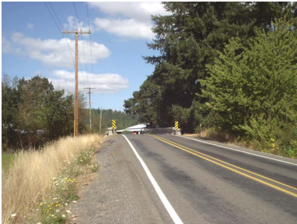
Photograph No. 6 — South bridge approach.
