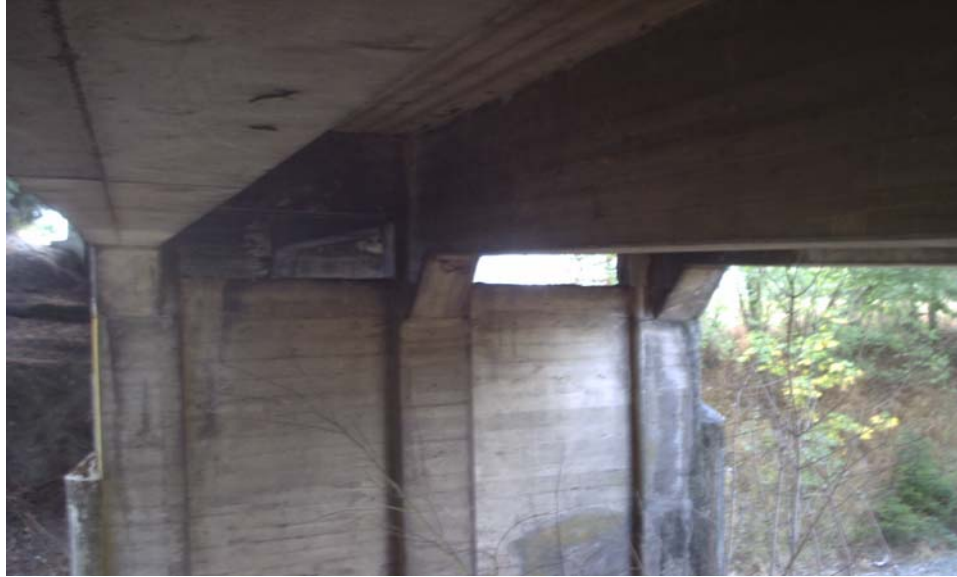
Photograph No. 3 — Bridge superstructure.
