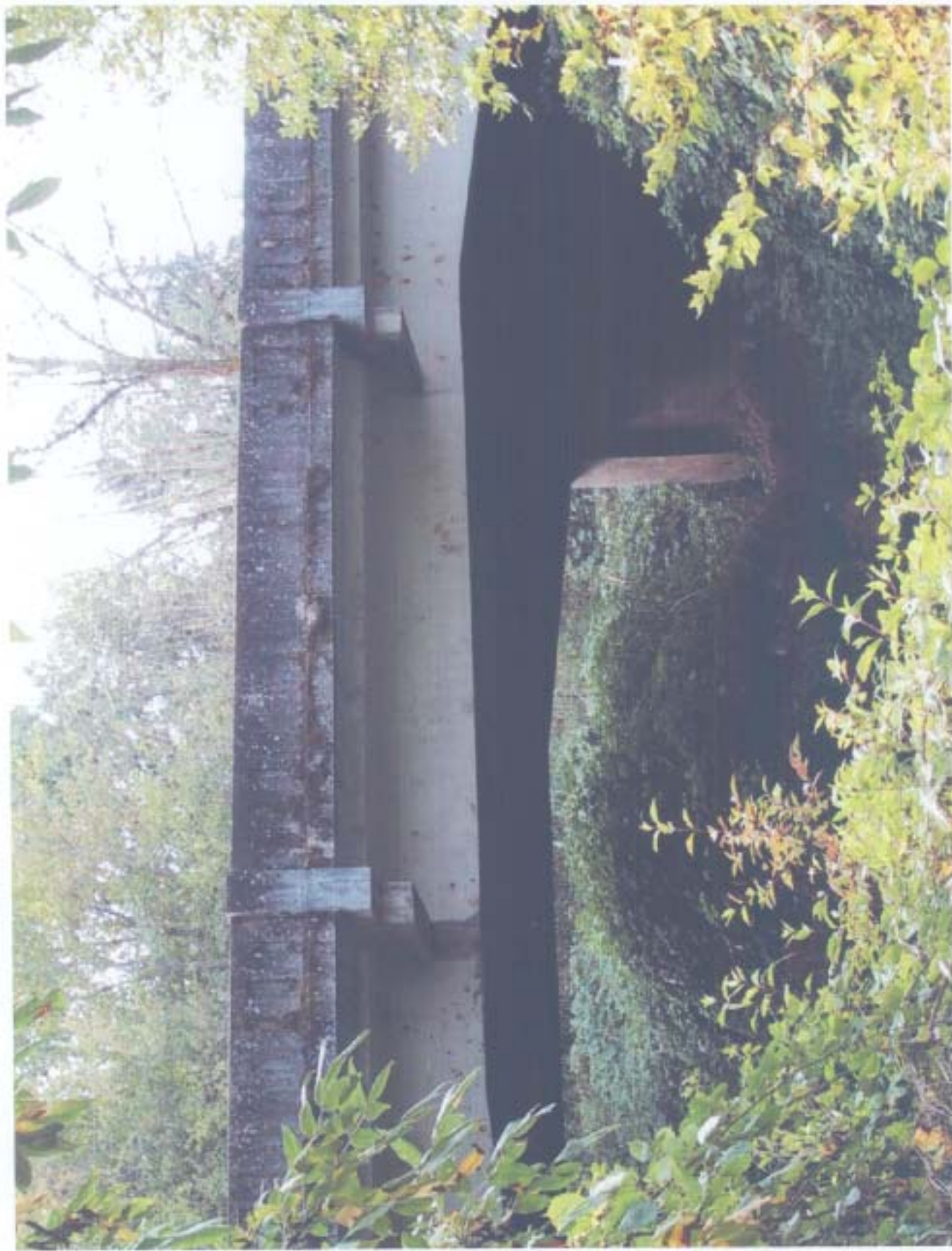
BRIDGE# 11540A BAKER CREEK. LOOKING UPSTREAM. (1600x1200x16M jpeg)
