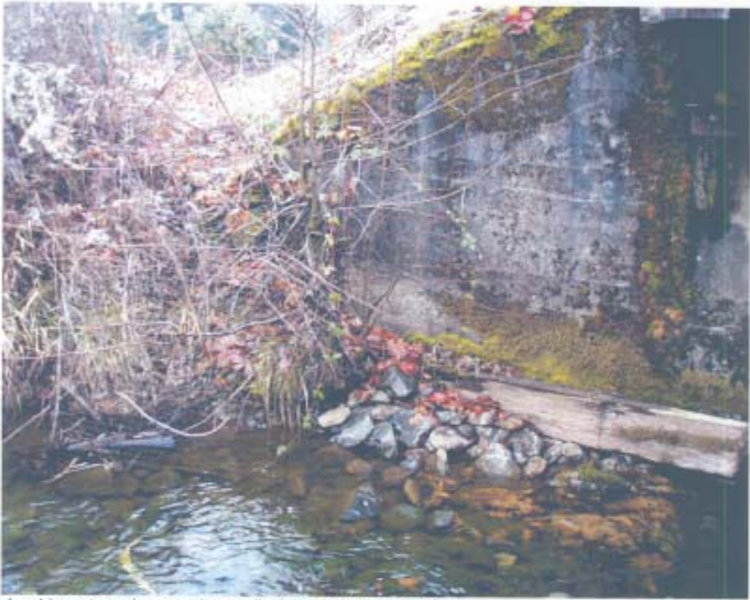
Looking at northwest wing wall of the north abutment.
