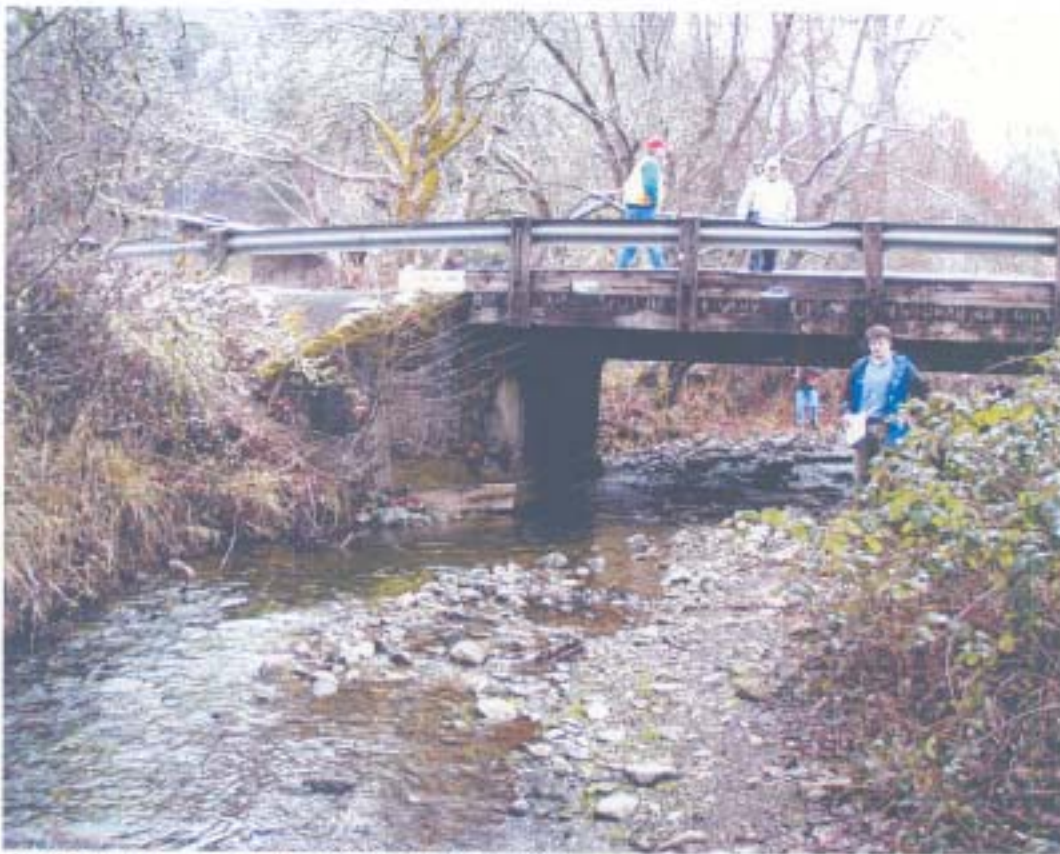
Looking east – upstream and at north abutment.
