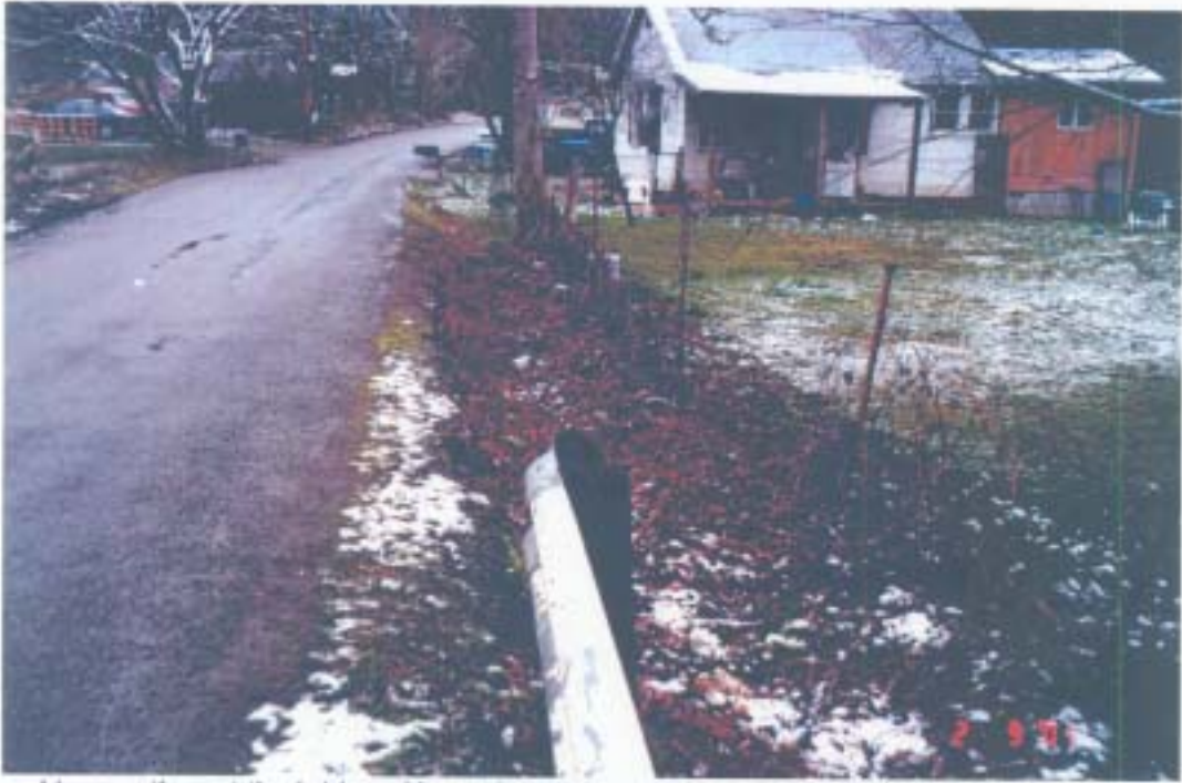
Looking south past the bridge. House located approximately 90 feet on west side.
