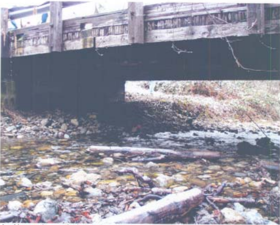
Looking south – south abutment.
