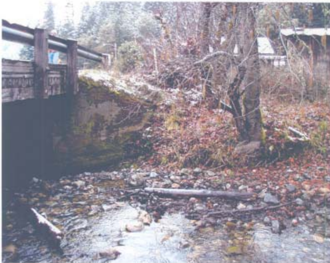
Looking north at northeast wingwall of the north abutment.
