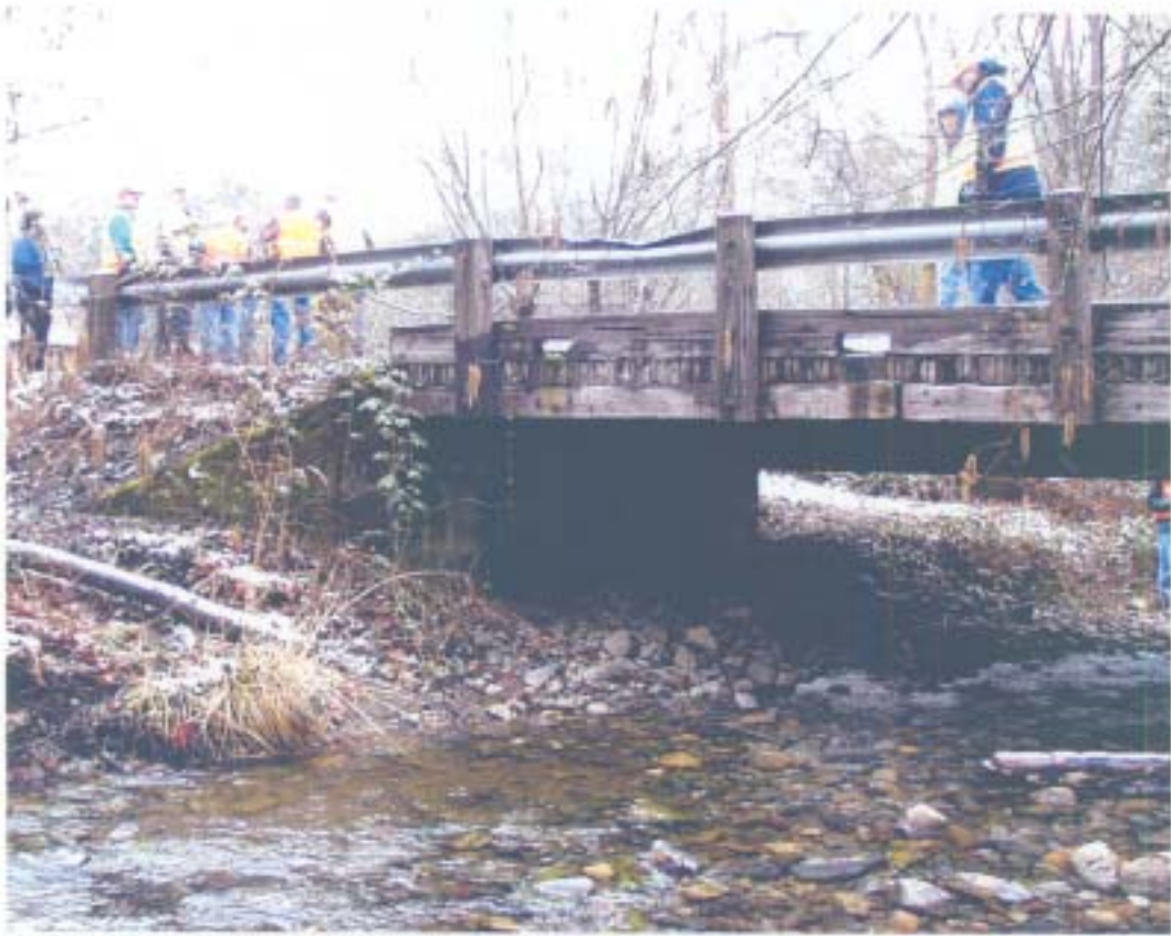
Looking south at the south abutment.
