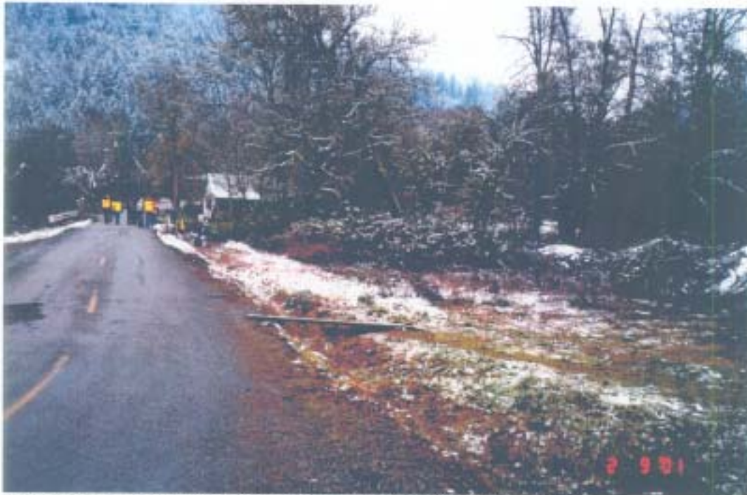
Looking south – ditch along west side of road and bridge in background.
