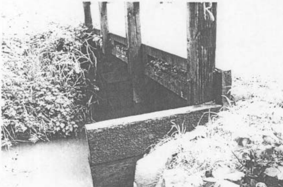
Looking ahead along left side.
