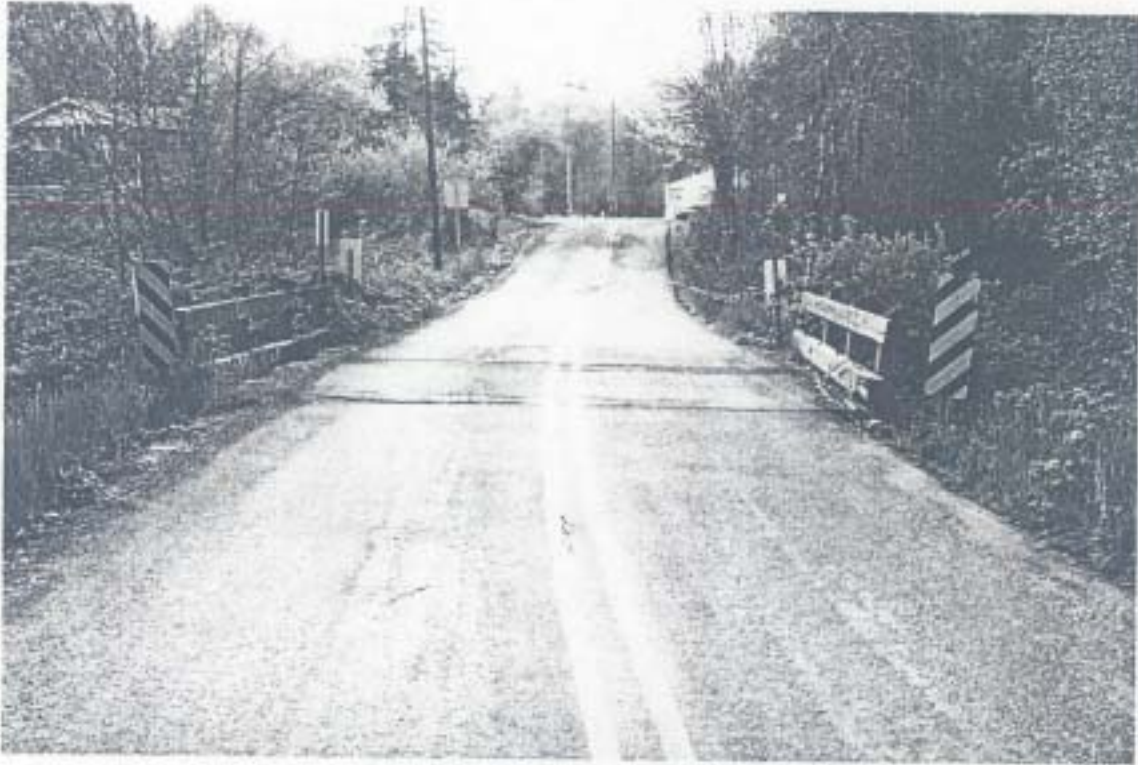
Looking ahead west.
