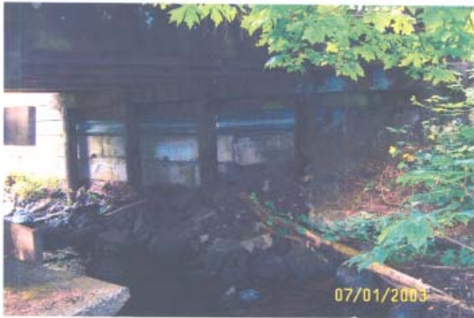
View of Backwall of Bent 3 repaired with concrete blocks
