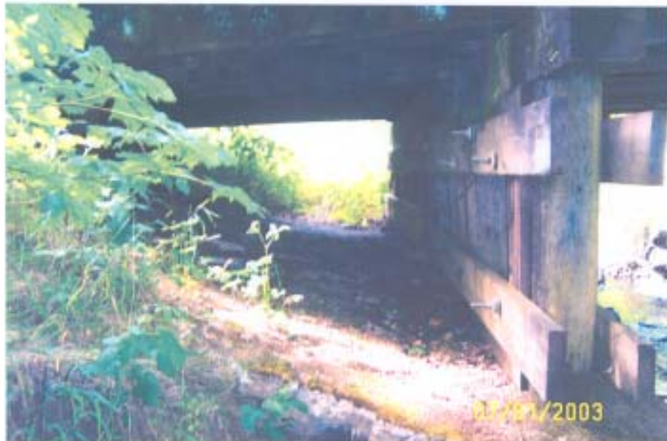
View of East Side of Bent 2 Fill was placed behind Bent 2 and covered with concrete for erosion control Fill has restricted flow through stream channel
